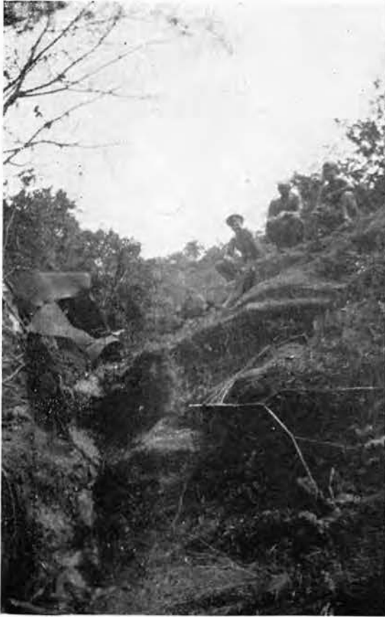
DYNAMITING OLD WATER DAM FIRST SOURCE OF WATER ON ISLAND
