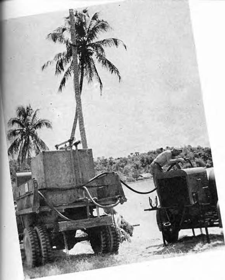
SEA-BEE MADE GASOLINE TRUCK REFUELING WATER PUMP
