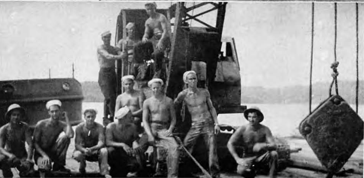
REPAIRING MAIN WHARF
