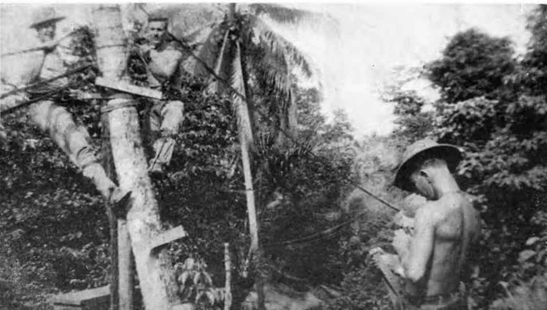
REPAIRING LINES IN JUNGLE
