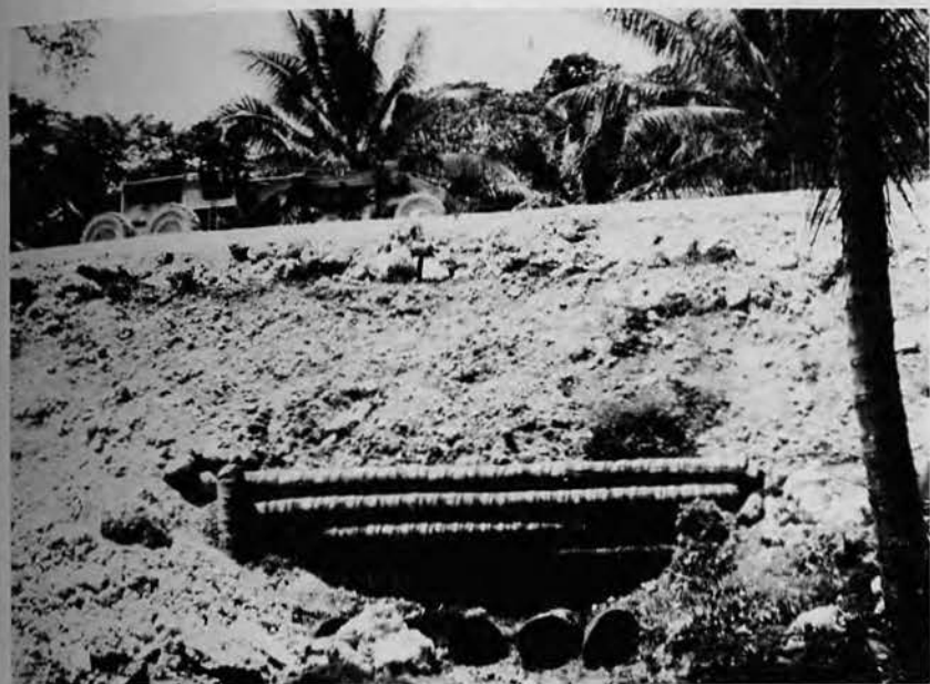
Above: Maintenance grader at work on section of roadway where drainage culvert has just been constructed. Five drainage pipes made of welded fuel drums. Below: A coral pit in operation.
