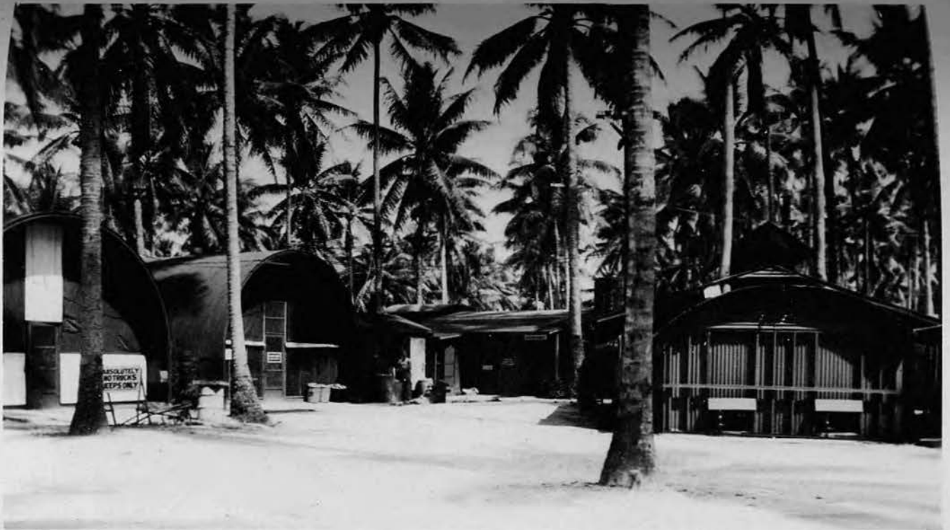
Camp galley area, showing (left to right) two commissary storage huts, including office in second one; refrigerator shack, galley entrance, and at right, bakery. Burners outside bakery heat two ovens, camp-constructed from pontoons. Entrance to one of enlisted men's two messhalls is partly visible at extreme right.
