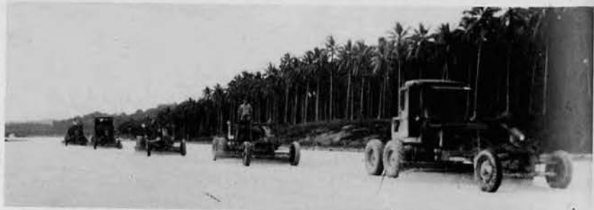
SCENES AT RENARD FIELD. Top: View showing Catalina flying boat and operational buildings of SCAT (Service Command Air Transport). Wimpy's Cafe behind plane. Center: Main strip. Control tower left center. Bottom: Graders at work on main strip.
