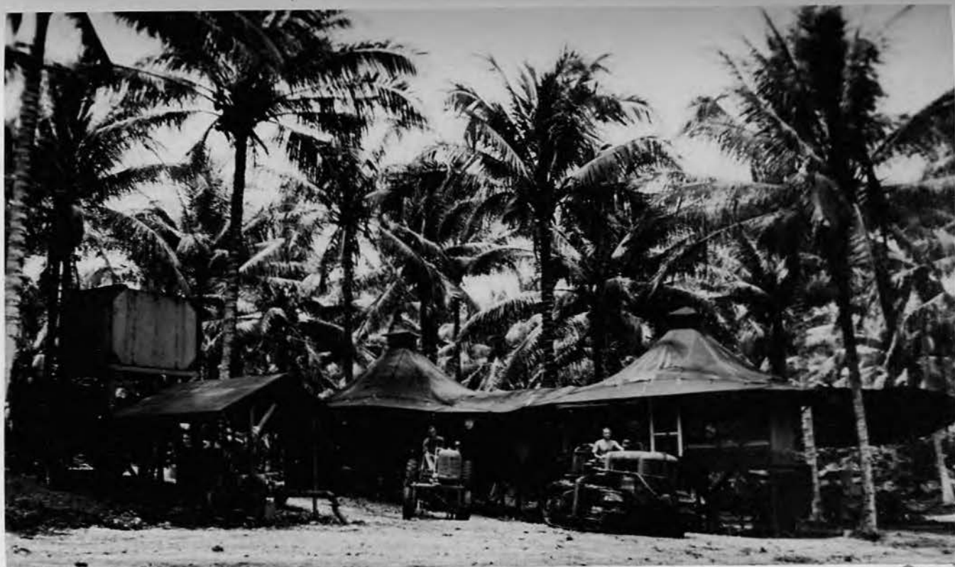
Quarters constructed at farm for farm workers. At left is water tank and pump. Galley and mess hall (center) is connected to sleeping quarters by sheltered companionway.
