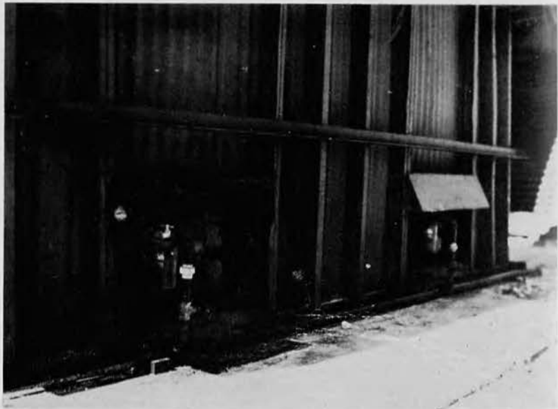
Bakery ovens built at camp from discarded pontoons. Top: Open view of one of two ovens, seen from interior of bakery. Bottom: Oil burner units for ovens, seen from exterior of Quonset hut bakery.
