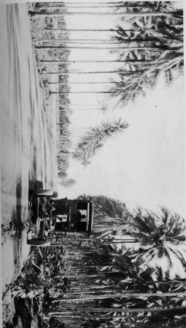
Road maintenance grader at work on section of South Massachusetts Boulevard near Marine warehouses and Blue Beach coral pit.
