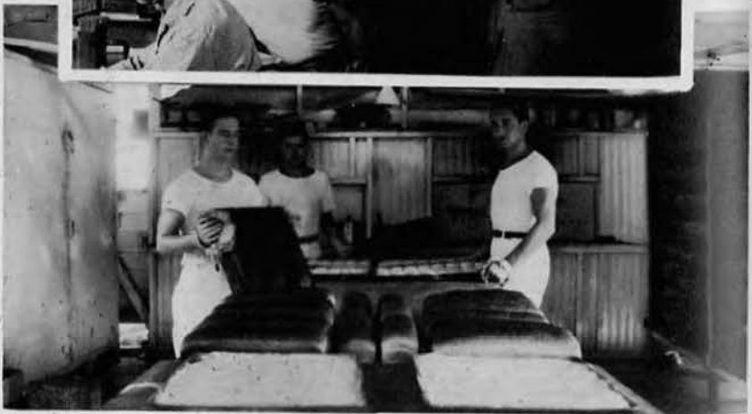
Top: Interior of Quonset hut camp galley. Center: Section of commissary office. Bottom: Interior view of camp bakery.
