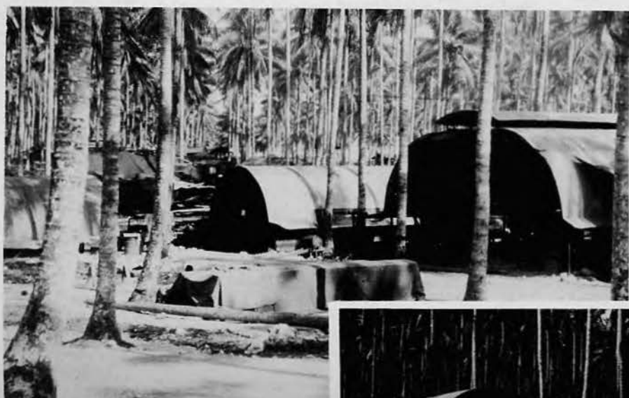
Right: Vehicle grease rack at left and fuel depot at right. Gasoline tank is made from pontoon. Quonset hut in background is carpenter shop.
