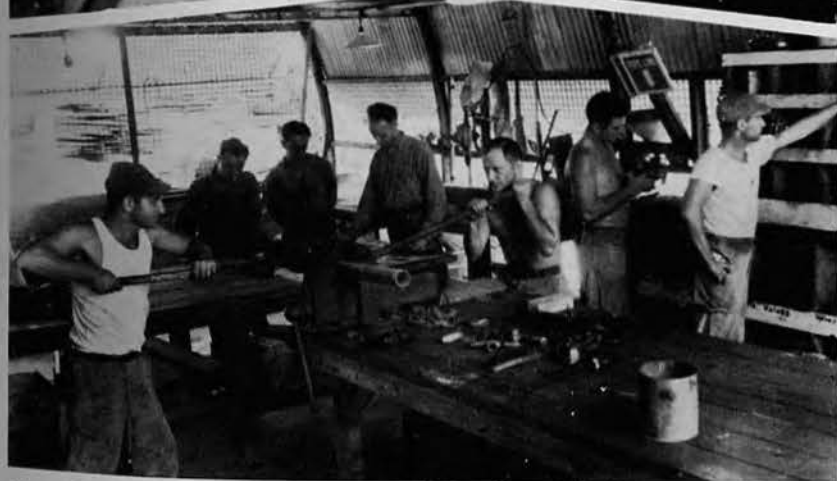
Upper left: Section of carpenter shop showing power saw in operation. Upper right: Welder at work in welding shop. Bottom: Plumbing, refrigeration and sheet metal shop.
