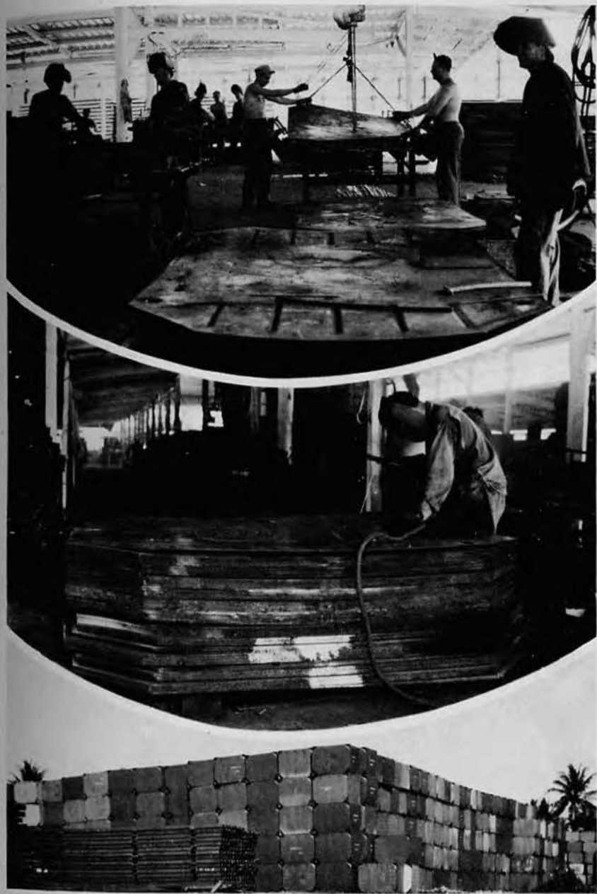
SCENES AT PONTOON ASSEMBLY DEPOT. Top: Prefabricated pontoon forms being set in place for welding. Center: Stack of prefabricated forms. Bottom: Piles of finished pontoons and connecting angles for stringing. Work shown here all done by PAD personnel. (Pontoon Assembly Depot No. 2 Photos)
