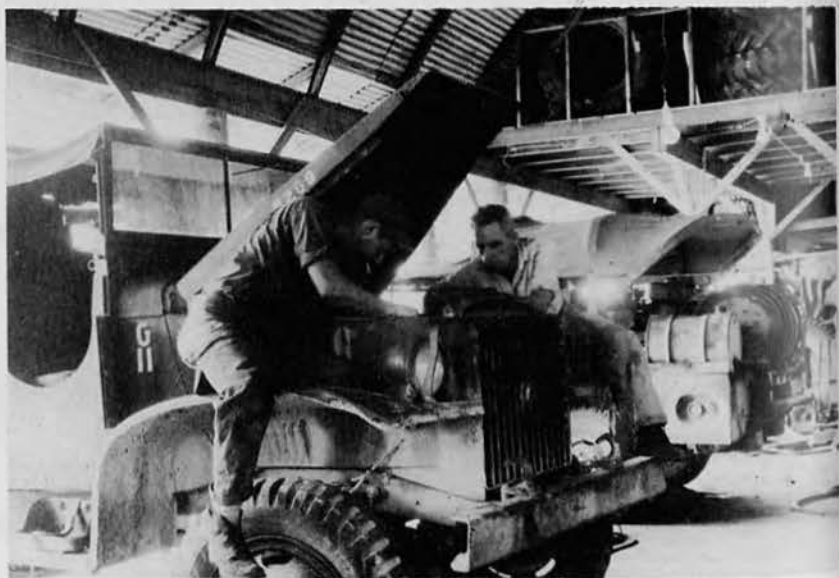
Above: Interior view of Quonset hut machine shop where many camp conveniences were contrived and manufactured besides other required items from lathe parts to surgical splints for battle casualties. Below: Motor overhauling at light equipment shed, showing tire loft and tire repair shop at right.
