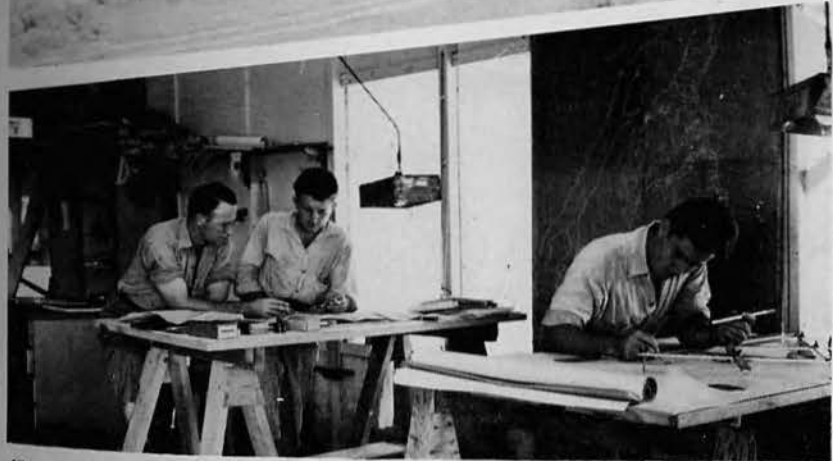
Top: Section of disbursing office in personnel building. Center: Exterior of personnel building, formerly plantation building. Bottom: View of drafting room located in wing of personnel building in foreground of center photograph.
