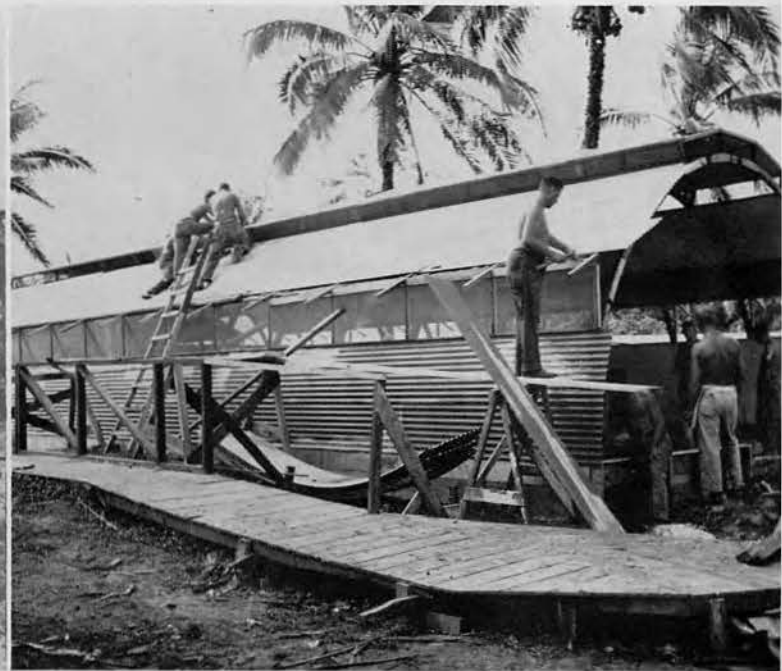
Physiotherapy ward under construction.
