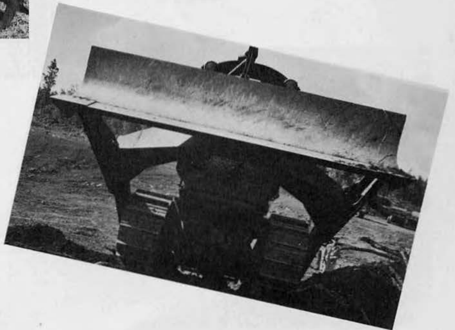
A heavy bulldozer lifts its steel snout over a volcanic hilltop.
