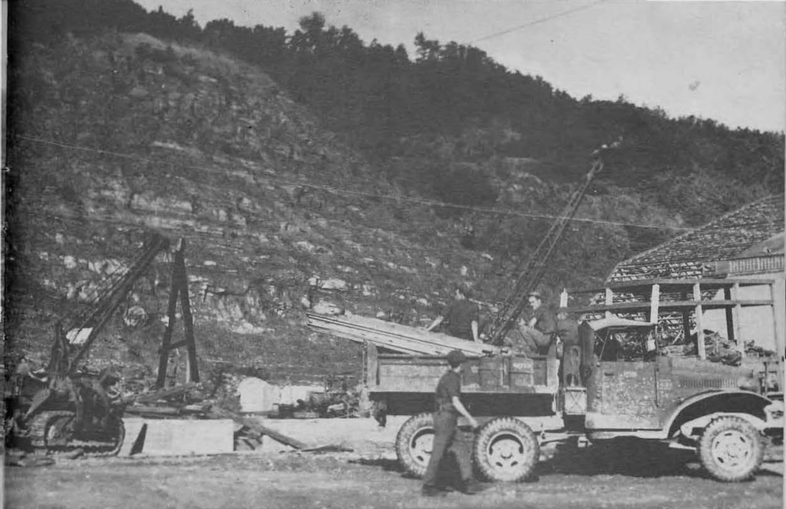
A construction battalion moves on its transportation facilities and does much of its important work with heavy equipment—so one of our first jobs was to clear an area for storage and maintenance.
