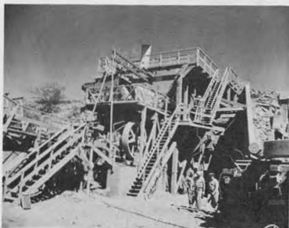
The stone taken from the quarry was crushed into usable sizes in the busy crusher operated by members of the battalion.
