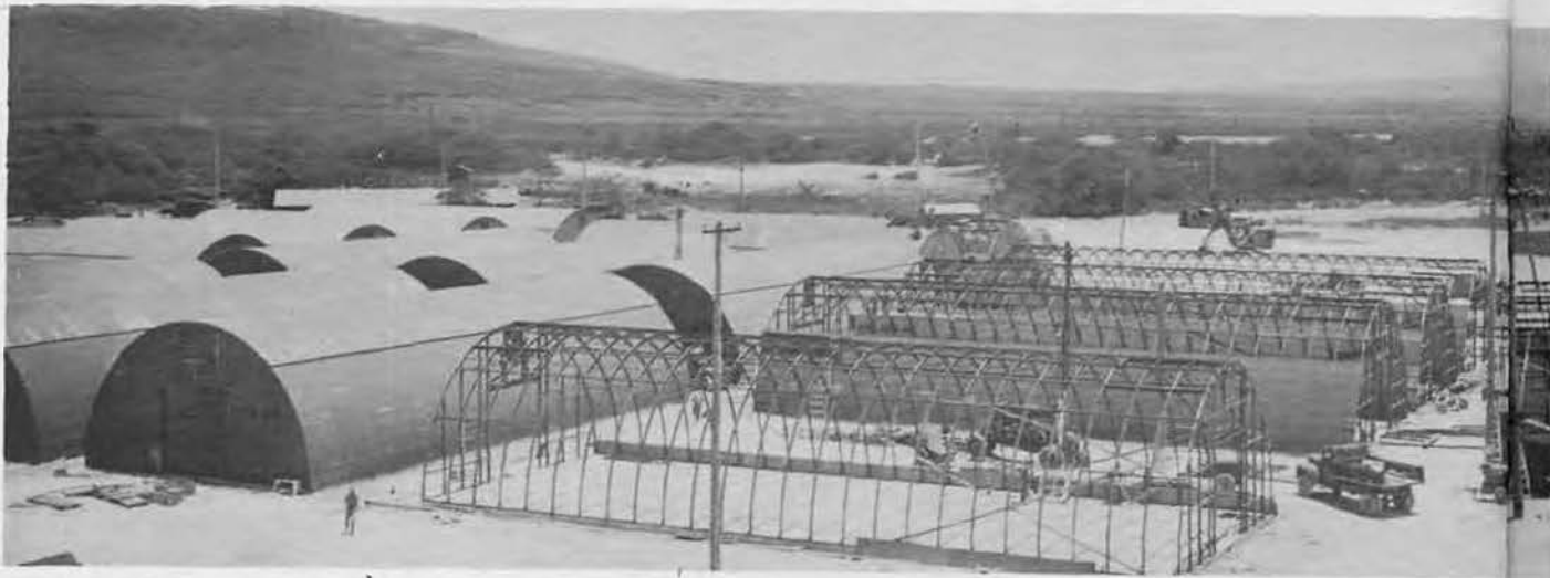
One of the largest and most important projects built by the battalion is the aircraft engine overhaul plant at a Naval Air Station, where battle-weary engines are renewed and returned to active duty. ABOVE: Quonset huts housing the plant were built on an assembly line basis, from laying the concrete slabs to putting the metal "skins" on the huts. BELOW RIGHT: As an adjunct to the overhaul plant, engine test cells for getting all "Bugs" out of the aircraft engines were built in record time.
