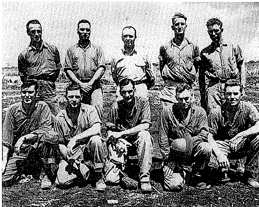
HUT ERECTION CREW
