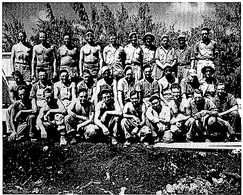
HOUSING AND FACILITY CONSTRUCTION CREW
