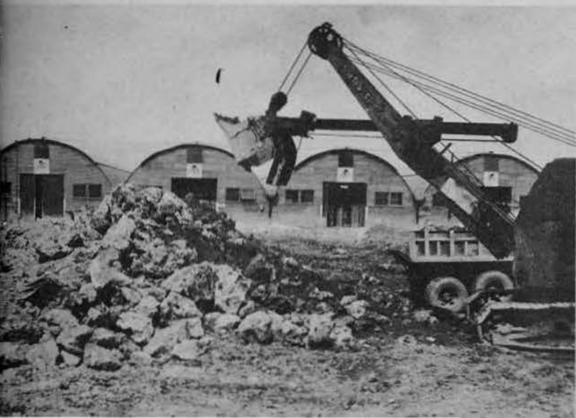
ROAD CONSTRUCTION PROJECT
