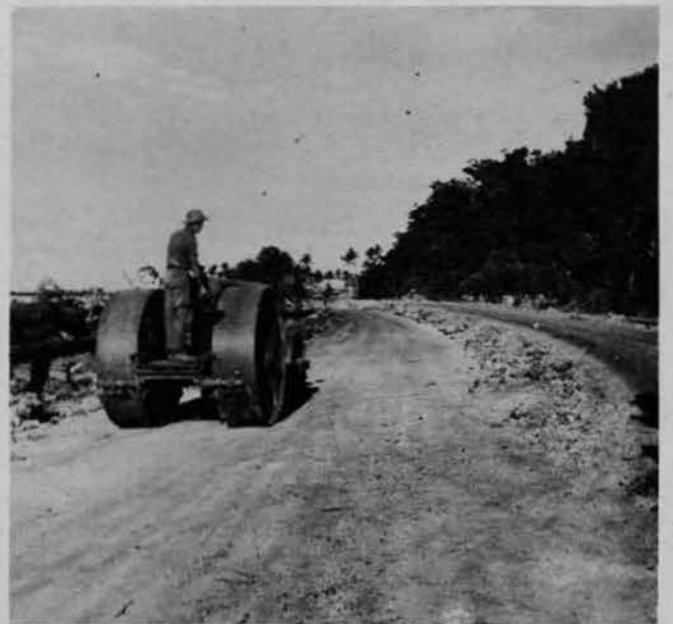
CALICOAN HIGHWAY CONSTRUCTION
