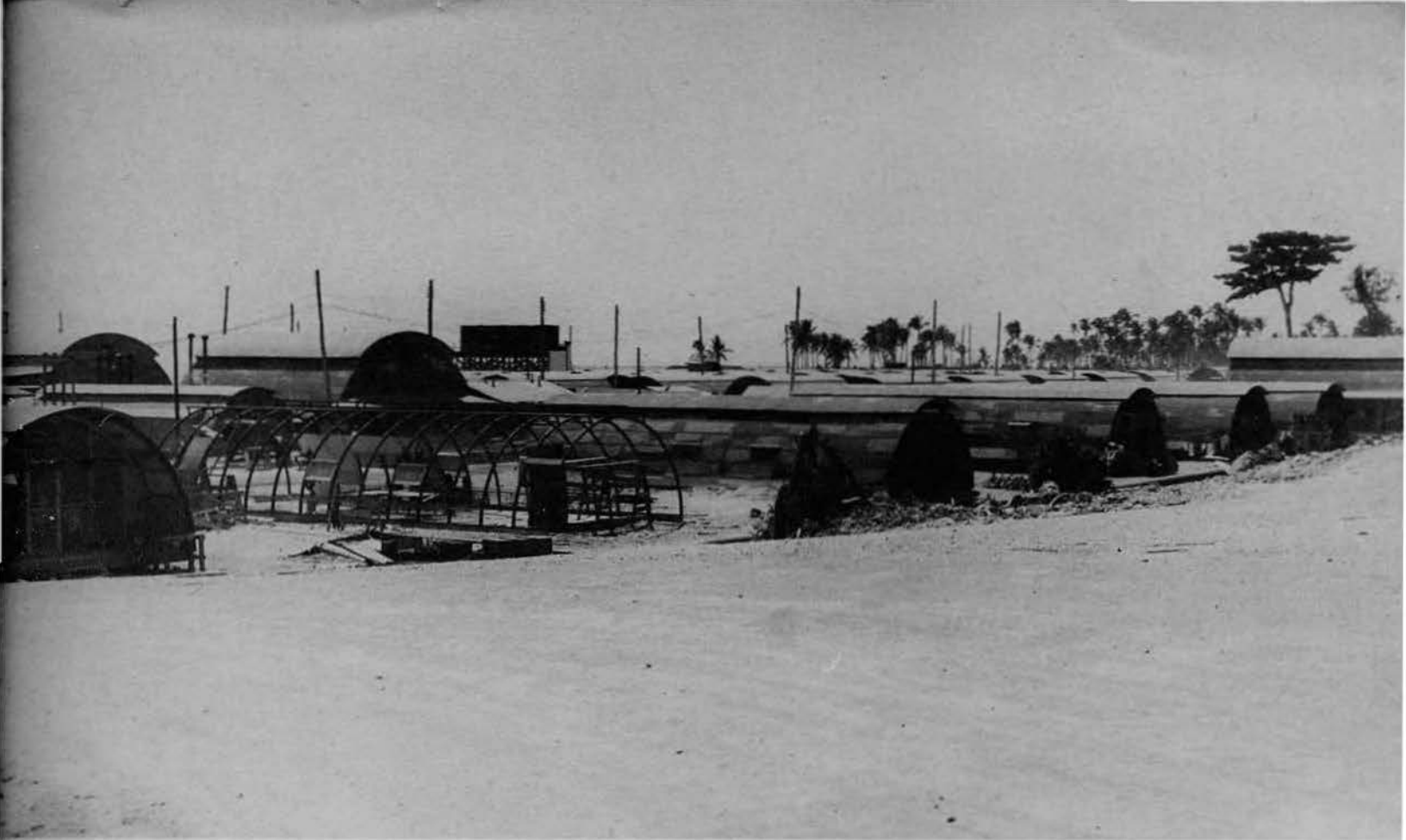
TWENTY-SIX HUNDRED MAN CAMP PROJECT
