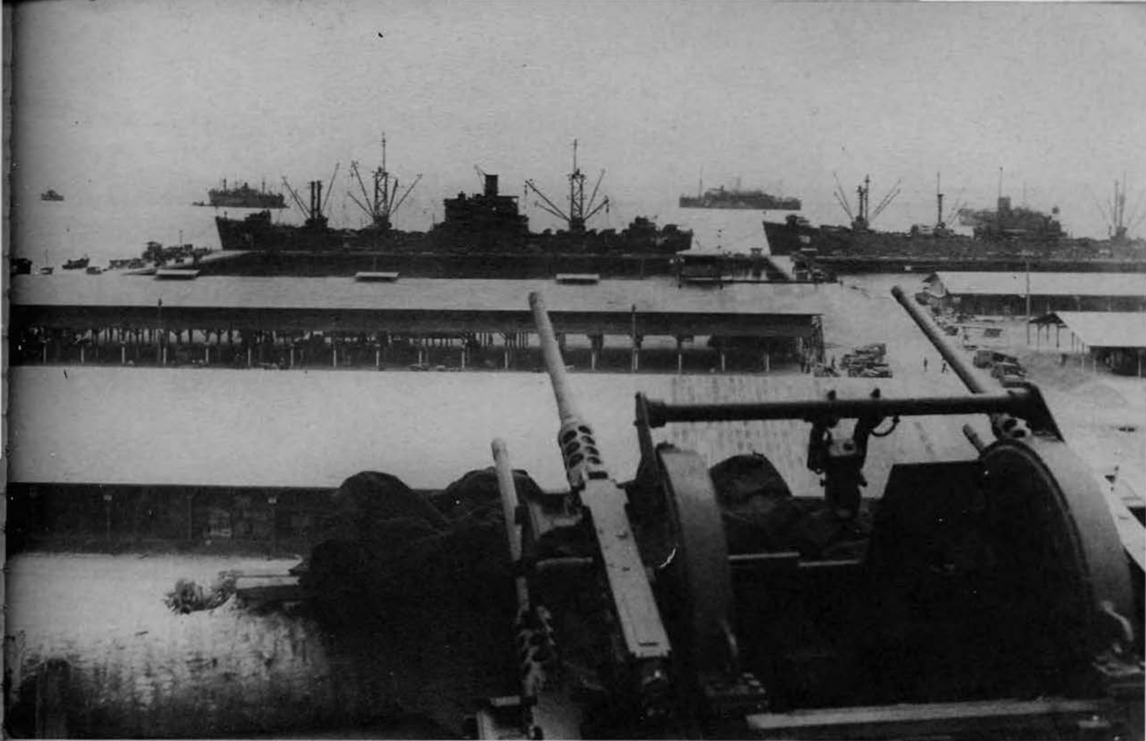
TWO STORY WAREHOUSE AND SORTING SHEDS PROJECT
