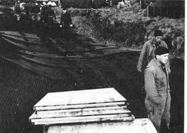
IF WE TRIED "beating a path" on the tundra we just sank farther in—so we pushed our wheelbarrows on metal mesh mats like these.
