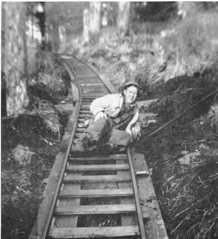
OVER HILLS and through forests we had to build our own narrow-gauge railway to transport supplies to our base far into the interior of the island.
