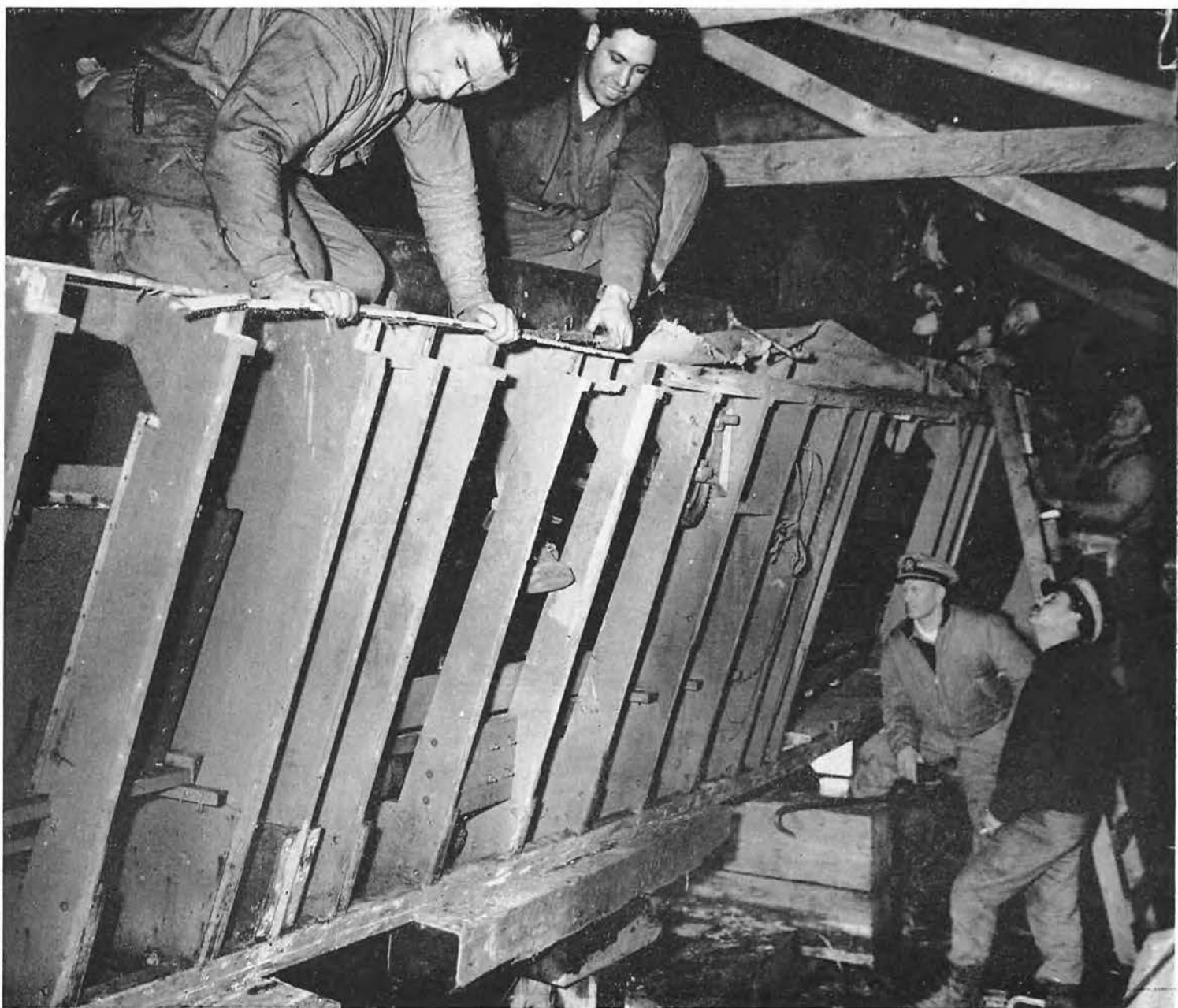
DURING the repairing process, we rebuilt the Higgins boat, baring its ribs and giving it new plywood sides. We built a new bottom, and slicked the 45th SEABEES
