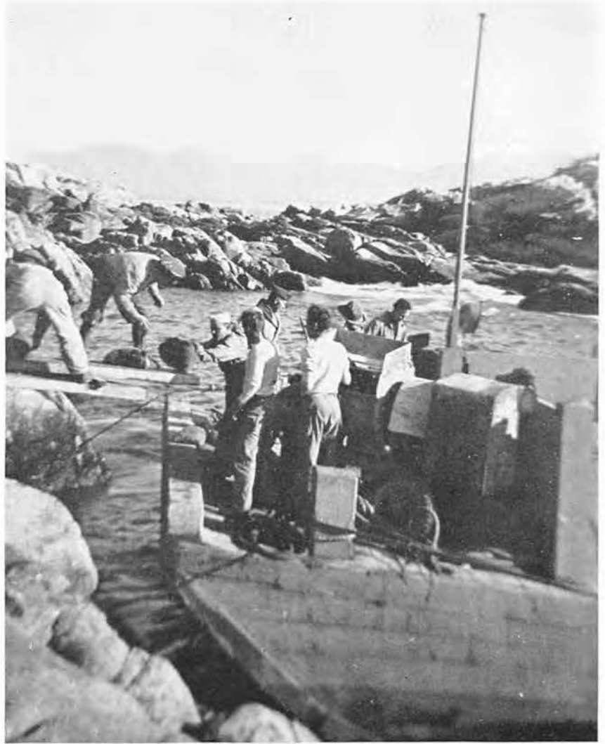
BY WATER WE CARRIED the "makings" which we later turned into strong concrete. Some spots were so inaccessible that water transportation was used exclusively.
