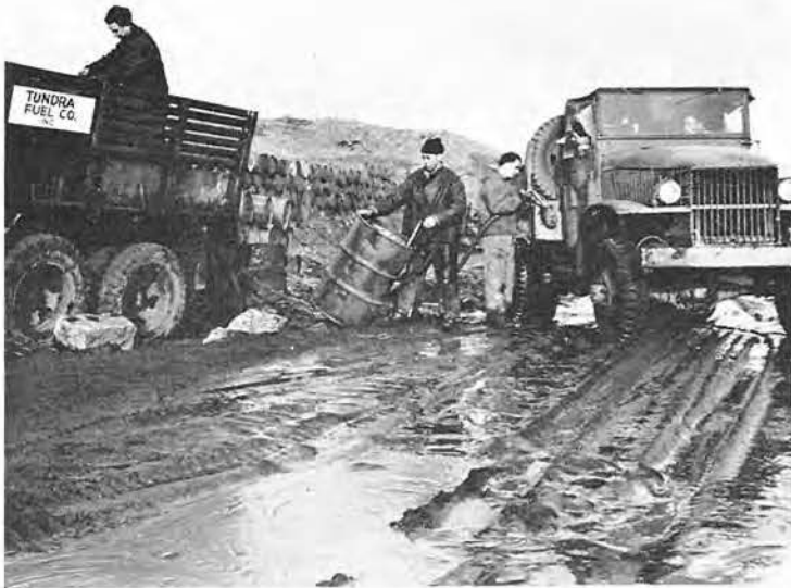
FILL 'ER UP —Aleutian style. Our filling station was mobile; if the truck couldn't get to the station, the station went to the truck.
