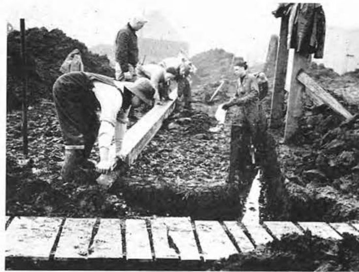
WHERE smaller pipes would do the job, we made them of wood. We scaped into the ditches as fast as we dug them.
