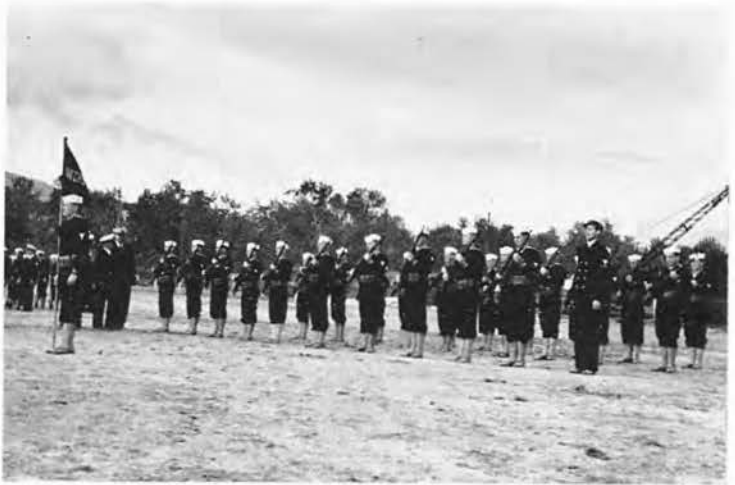
HEADQUARTERS COMPANY men present their rifles, bolts open, for inspection.
