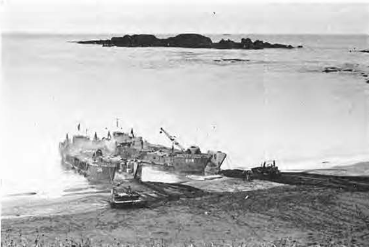
LONELY LOOKED the beach, and empty, that first morning, as bulldozers bit into the sand and built ramps for unloading the LCT's.
