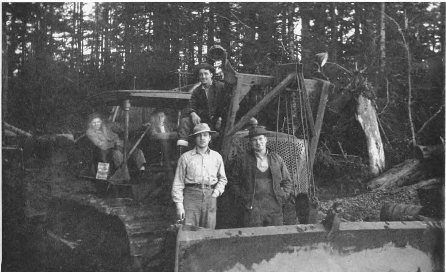
WITH BULLDOZERS we pushed our way through the primitive forest beds when the timber had been cleared away. It was the first time much of the virgin soil had ever been touched with the blades of modern machinery.
