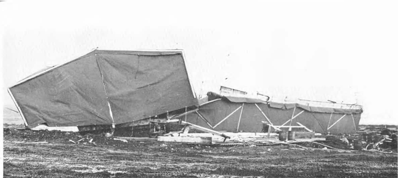
A WILLIOW one night picked up our machine shop and set it down again. The section at the right was turned upside down in the process. Later we
