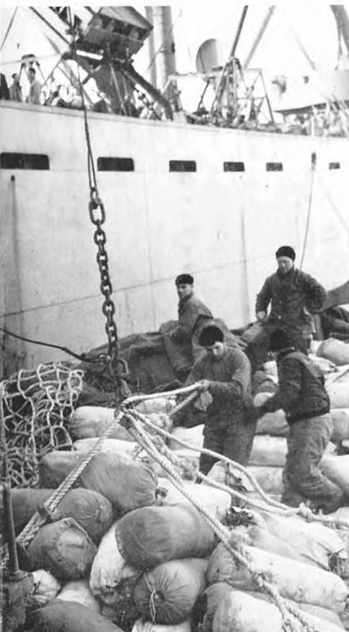
WHAT WE couldn't carry, we hoisted aboard in a cargo net. We loaded all the cargo on this Liberty ship from dock to barge, barge to ship.
