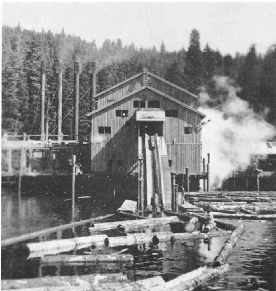
SOME OF THE LUMBER AND TIMBER used in our construction work was cut near our base from trees felled in the neighborhood. Usually there was water enough around us to make transportation of the logs an easy problem.
