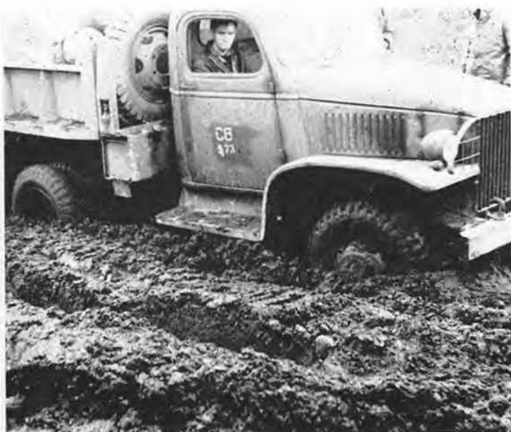
BEFORE the sand was put on, heavy trucks mired hub deep in the mud. This is the way the tundra looked when the top layer was scraped off.
