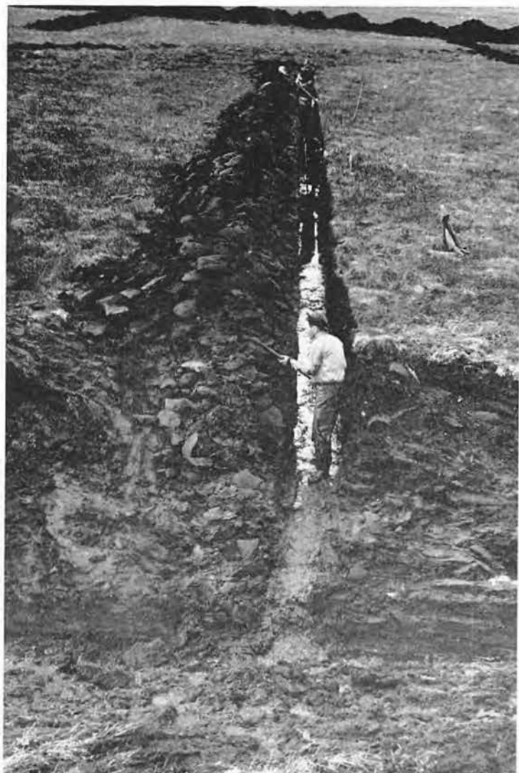
HAND-DIGGING of ditches with a "Japanese dragline" or "idiot stick" wasn't very glamorous, but it was a vitally important part of the job.
