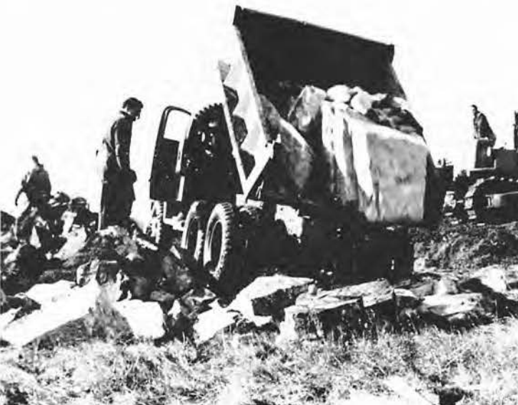
WE USED ROCKS FROM OUR towering quarry to lay a foundation for our roads. Gradually, though, the rocks sank deeper and deeper.
