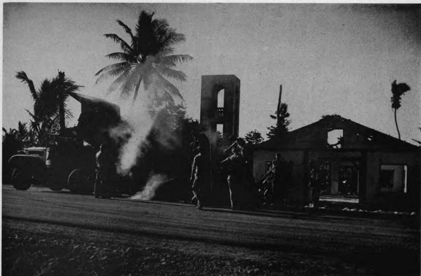
Above: Black-top spreader gang laying a modern asphalt pavement!
