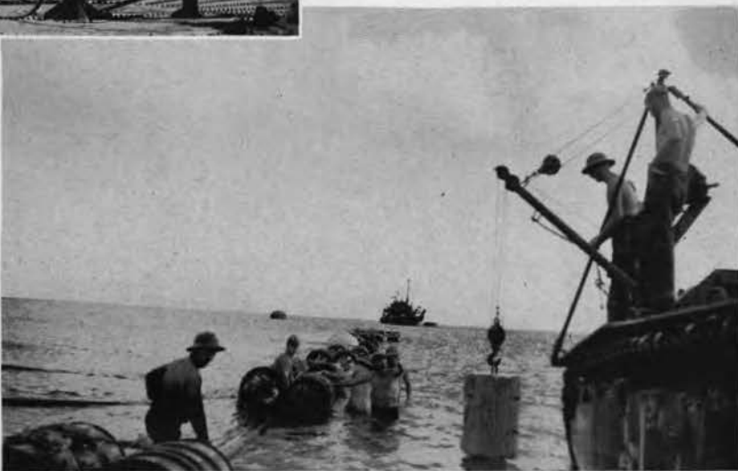
Above: Laying the second ring on gasoline storage tank.
