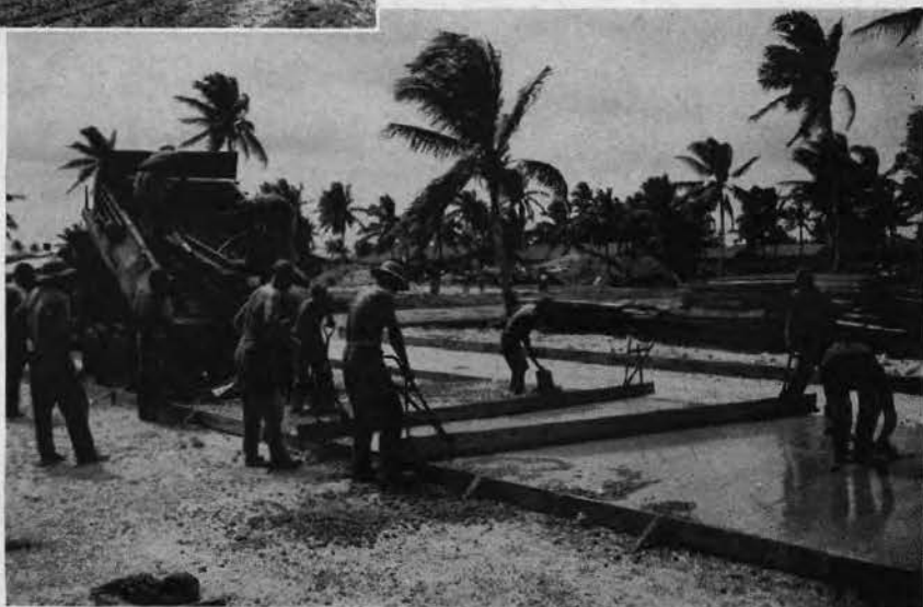
Below: Concrete finishers. Note the improvised 'b a t c h' truck!
