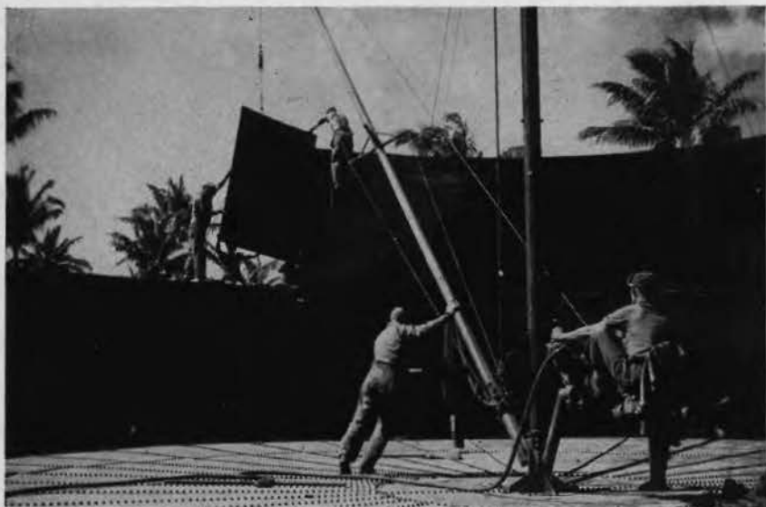
Above: Laying the second ring on gasoline storage tank.
