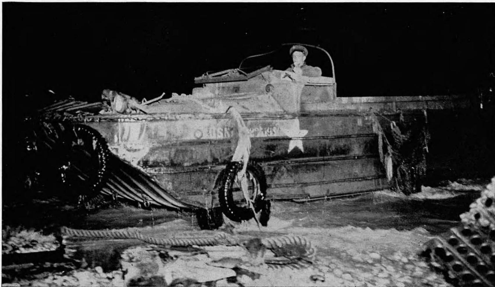
FERRY DUCK: Operated as a personnel and supply carrier between the beach and the Rhino repair barge.
