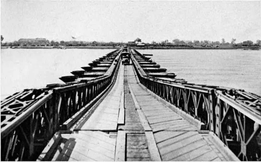
BAILEY BRIDGE installed across the Maas River.
