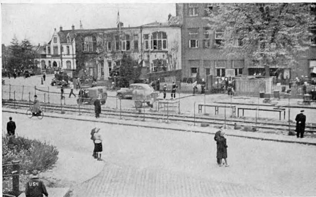
TASK FORCE BILLET in the former office building of the Stork Machine Fabrik at Hengelo, (O), Holland.
