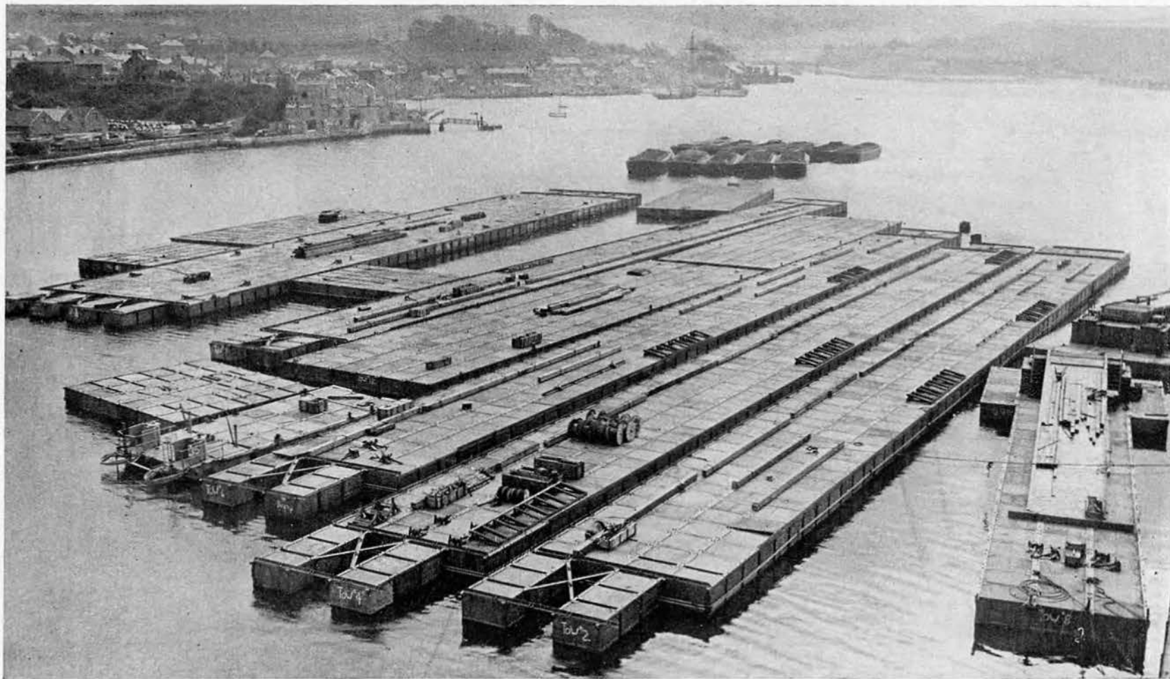
ASSEMBLED TOWS lying at anchor near Cattedown Wharves, Plymouth. Paraphernalia distributed on decks is for use in the installation of the piers.
