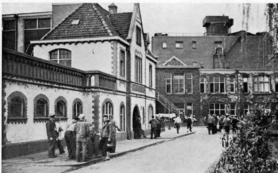
BATH HOUSE AT HENGELO was pressed into service to take the bathers off the streets and away from the public gaze.
