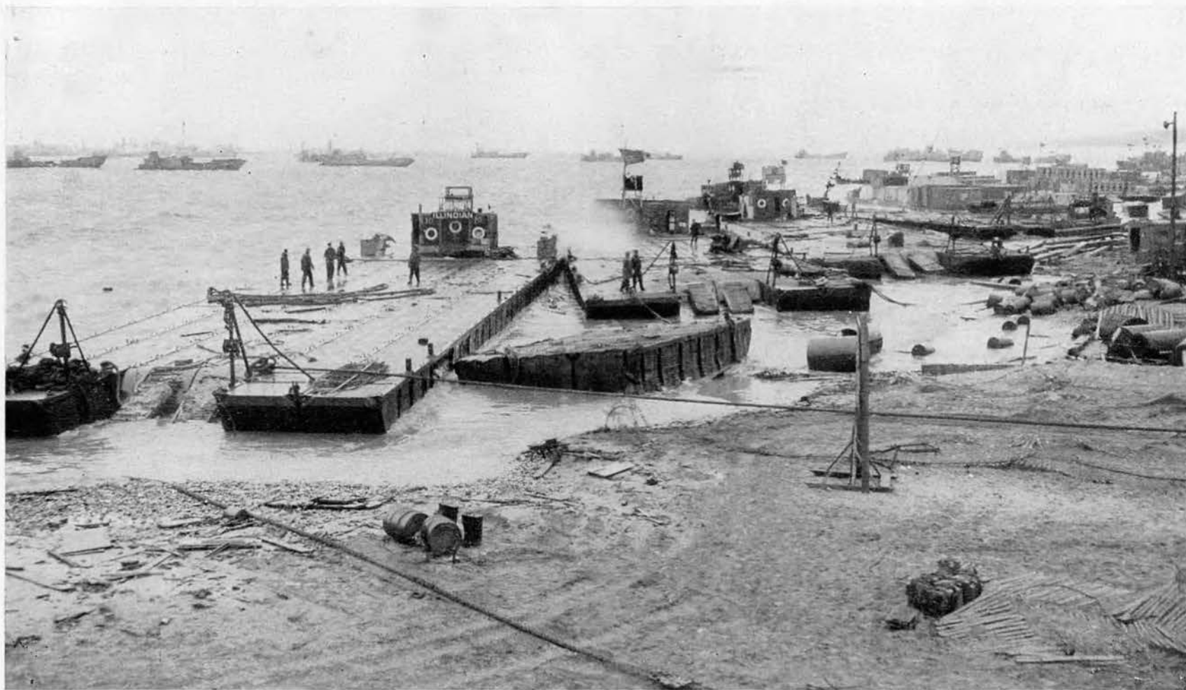
AFTERMATH OF STORM that closed Omaha Beach as an operational port. Huge swells breaking over the blockships cast Rhinos and other craft high on the beach, causing critical damage.
