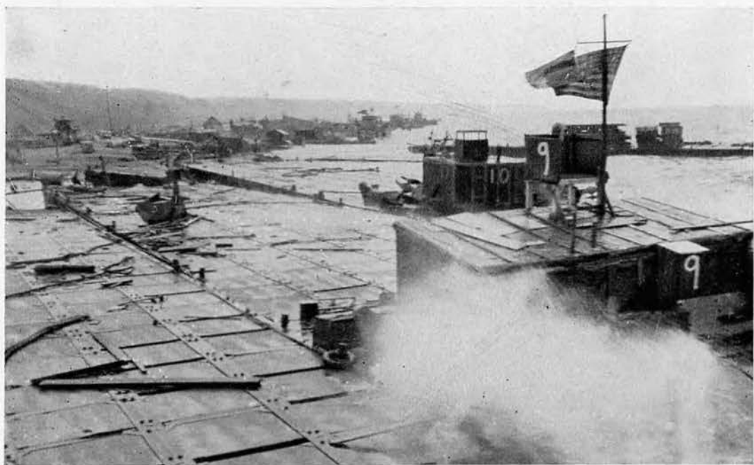
BREAKERS WASHING THE DECKS OF RHINOS as they pound and grind together on the beach.
