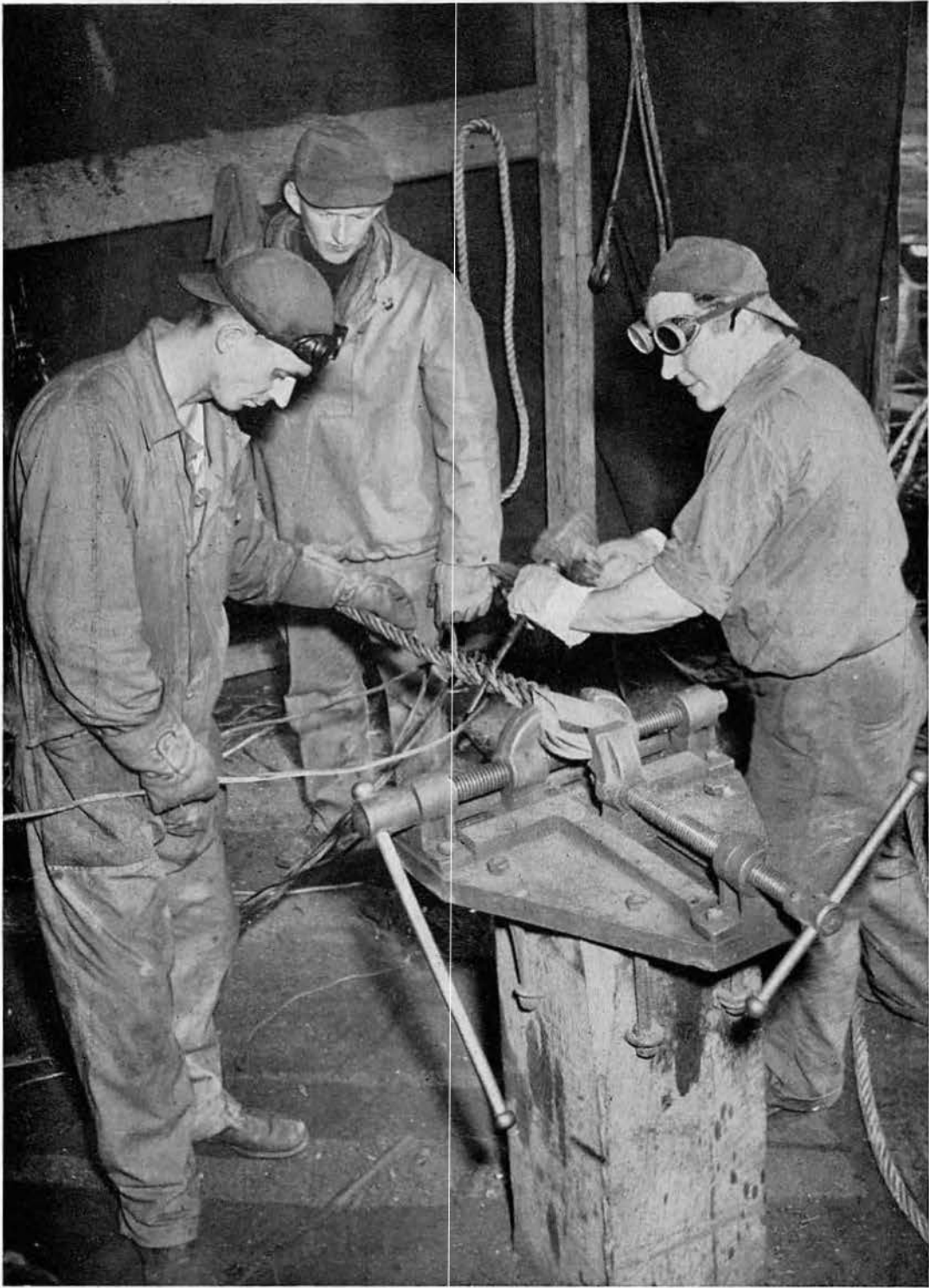
TOW BRIDLES: Riggers splicing a thimble into a heavy cable to be used in harnessing the tows for delivery to destination.
