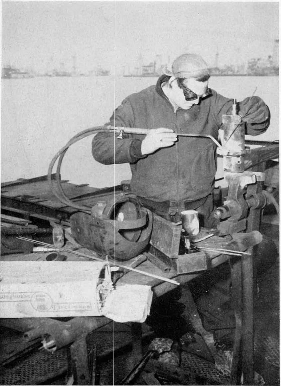
BRAZING: Broken parts must frequently be retained in service. Welders keep busy in maintaining equipment not easily replaced.
