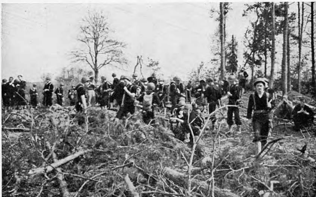
ARRIVAL AT THE SITES: Demolition charges had shattered the dense pine woods and woodcutters had moved in to salvage the timber for firewood.
