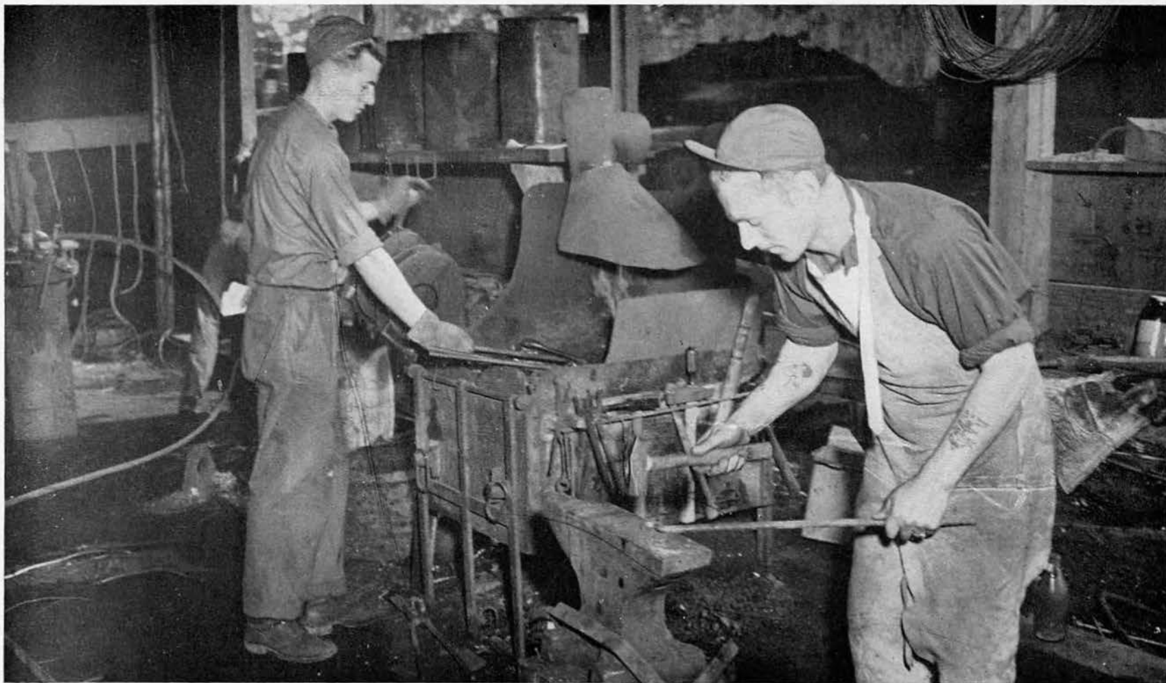
BLACKSMITH SHOP: Expansion of pontoon assembly operations created a demand for "jewel wrenches", an improvised tool. Blacksmiths heat and shape them.
