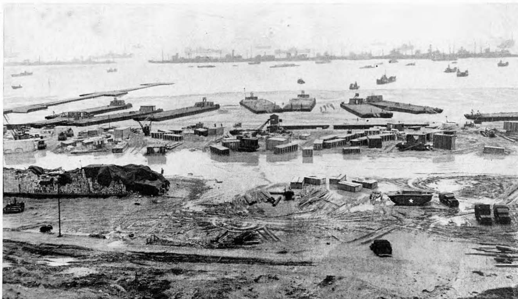
OMAHA BEACH: Scene of operations. Sunken blockships in background with troop and supply ships anchored beyond. Left center, the sunken causeway. Center, Rhino Barges "dried out" on beach at low tide, and in foreground, equipment and supplies ferried ashore by Rhinos.
