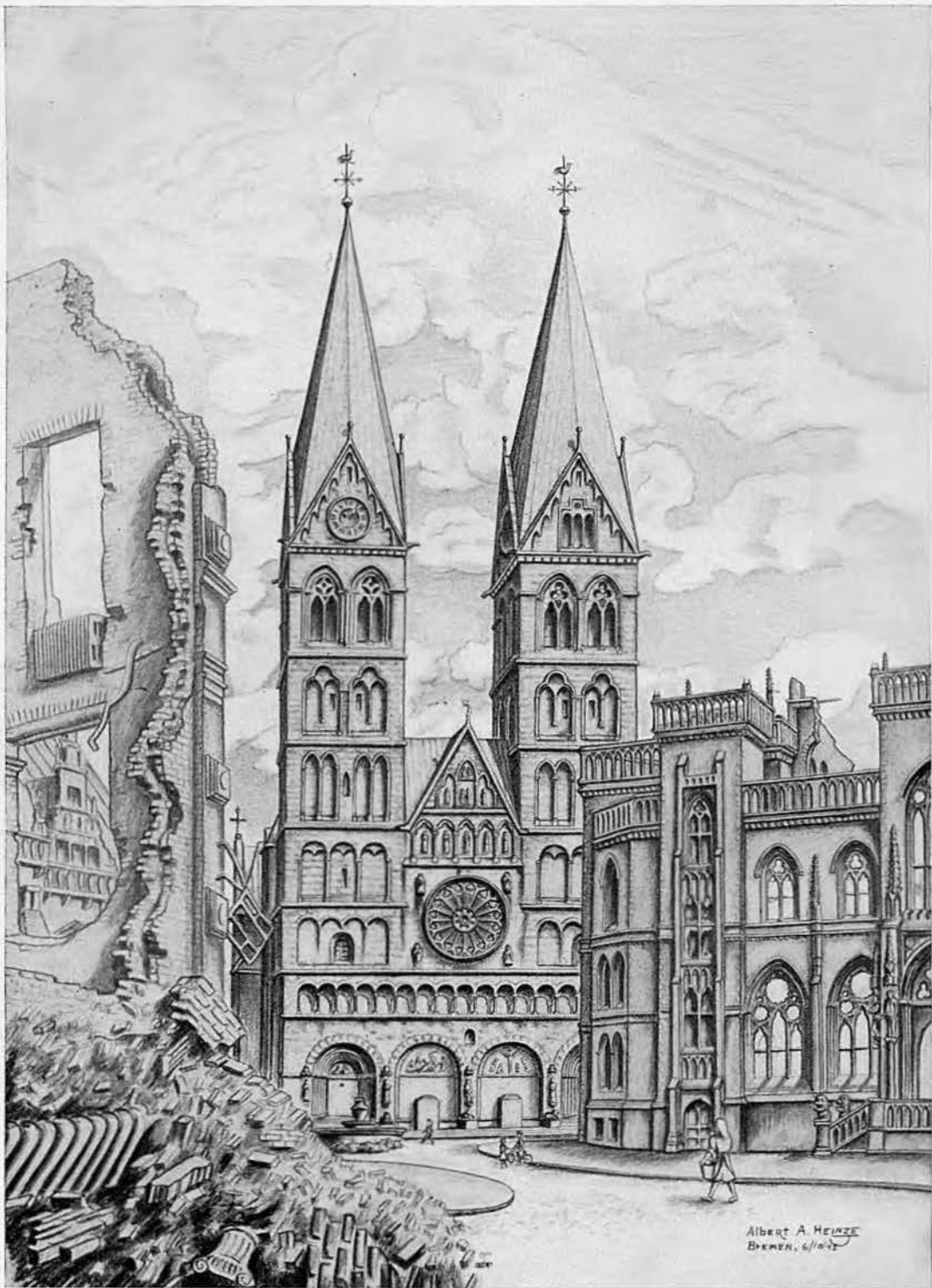
THE BREMEN DOM. The erection of St. Petri Cathedral on the Marktplatz began in the early medieval period 1003 A.D. but was not completed in present form until the late 19th century. Dom and the Bosse at right were damaged in air raids of October 1944.
