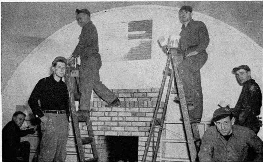
PAINTERS working on one of the many paint jobs assigned the Sixty-Ninth throughout England. This job — Hamoaze House.
