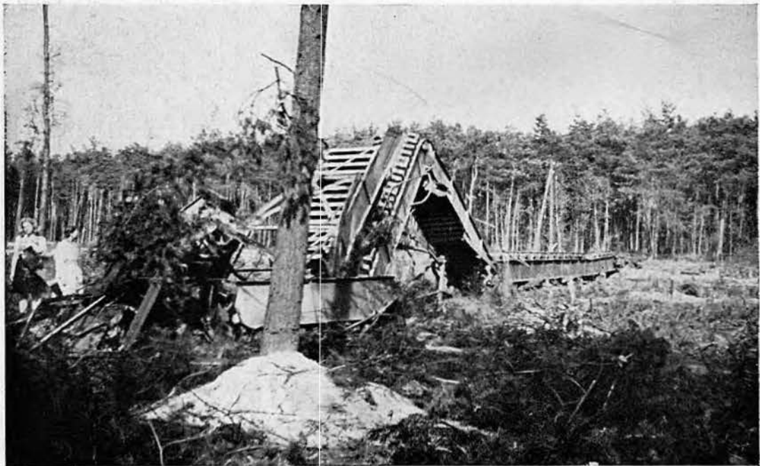
DEMOLITION CHARGES set off by the operating crews before abandoning the sites prostrated the catapults as shown.
