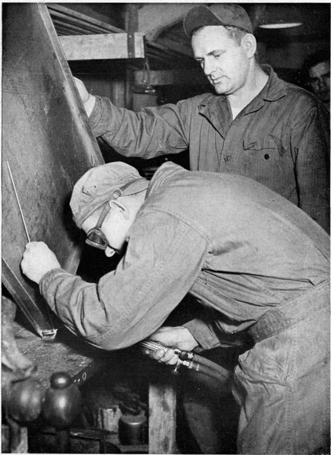
METALSMITHS engaged in maintenance work, braze an angle at Vicarage Camp.
