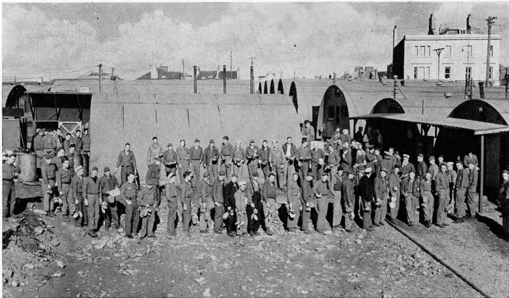
CHOW AND SCULLERY LINES: Personnel returned to Edinburgh Road Camp temporarily, after false start for France. Delay was caused by rough water in the channel.
