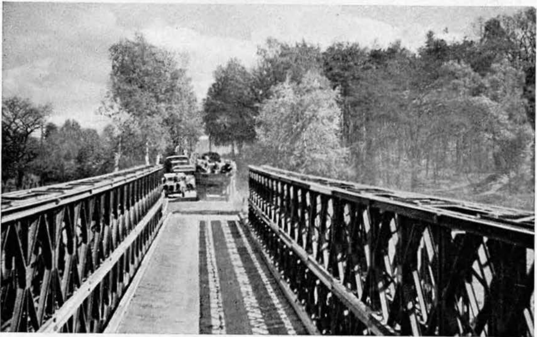
BAILEY BRIDGES replaced all the bridges the retreating Wehrmacht destroyed in its effort to stem the Allied advance across the British sector.
