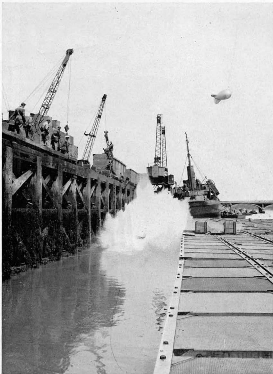
A LAUNCHING SEQUENCE to the previous picture of the completed strings. Such "shakedown" as this, occasionally necessitated the retightening of bolts, loosened by the impact.
