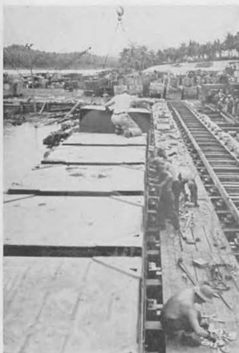
Placing T-6 pontoon
