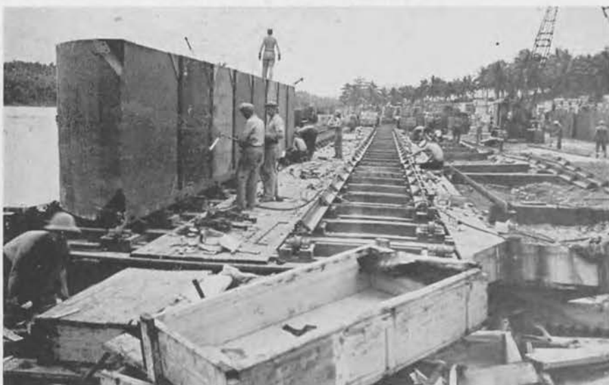
Burning hole for bolts
