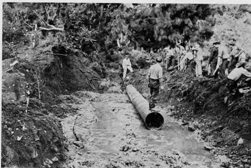
Digging drainage ditch
