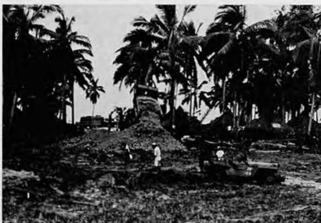
Fill-in galley area
