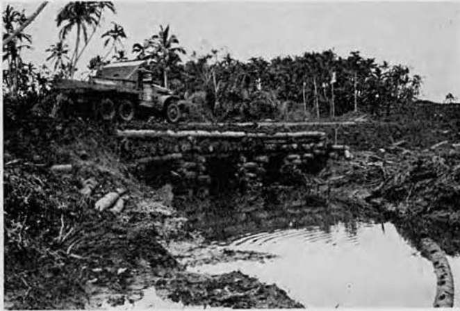
Bridge over drainage ditch
