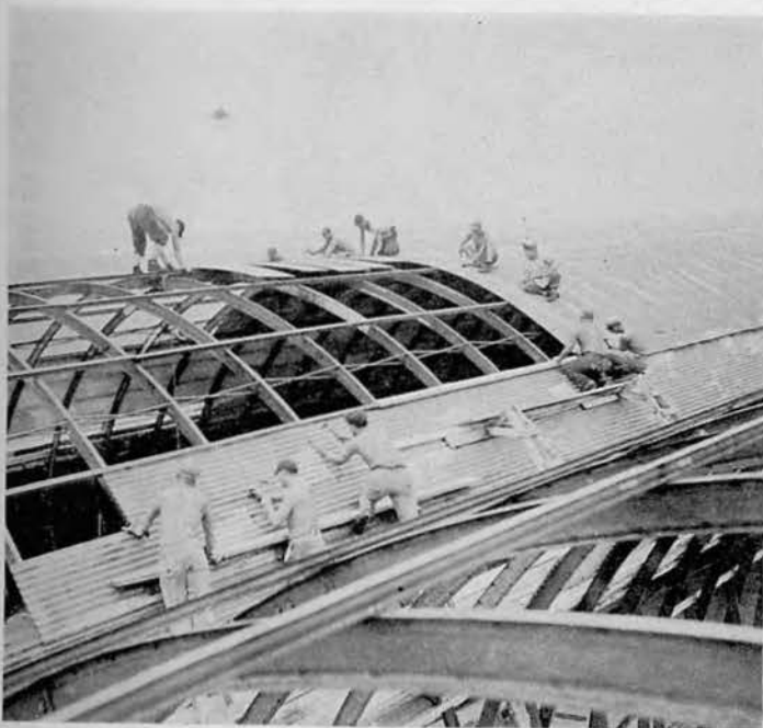
Quonset Hut Erection
