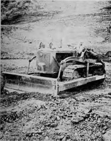
Grading for dock
