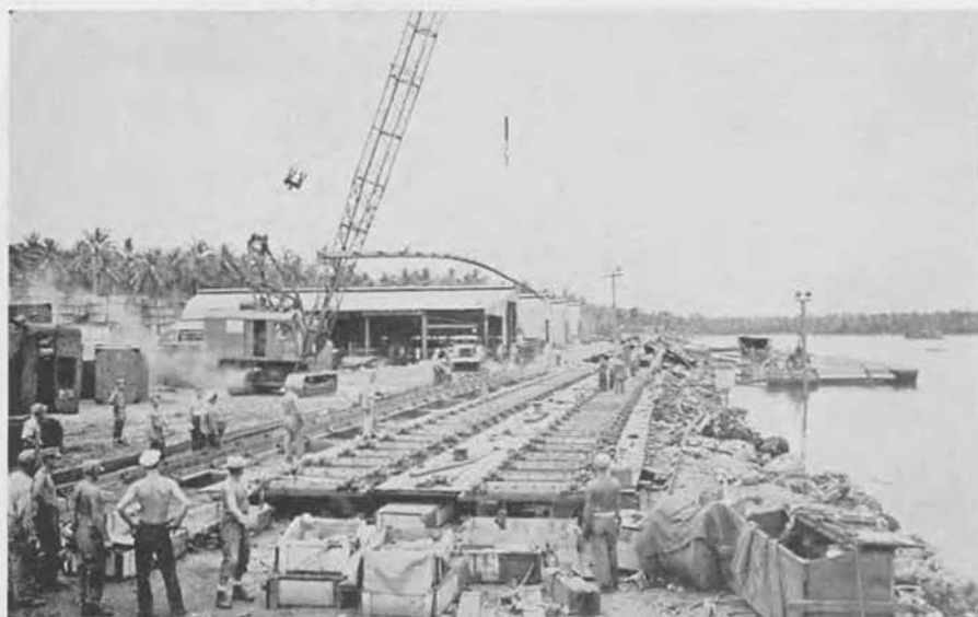
B-11 angle coming in position
