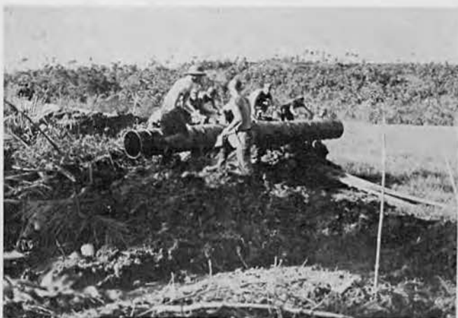
Culvert laying
