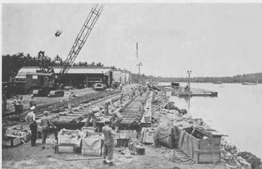
Angle placed and bolts ready
