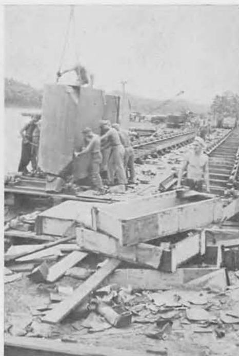
Placing P-7 pontoon
