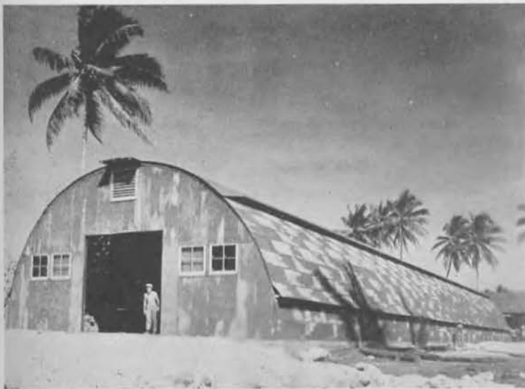
Fill-in around hut
