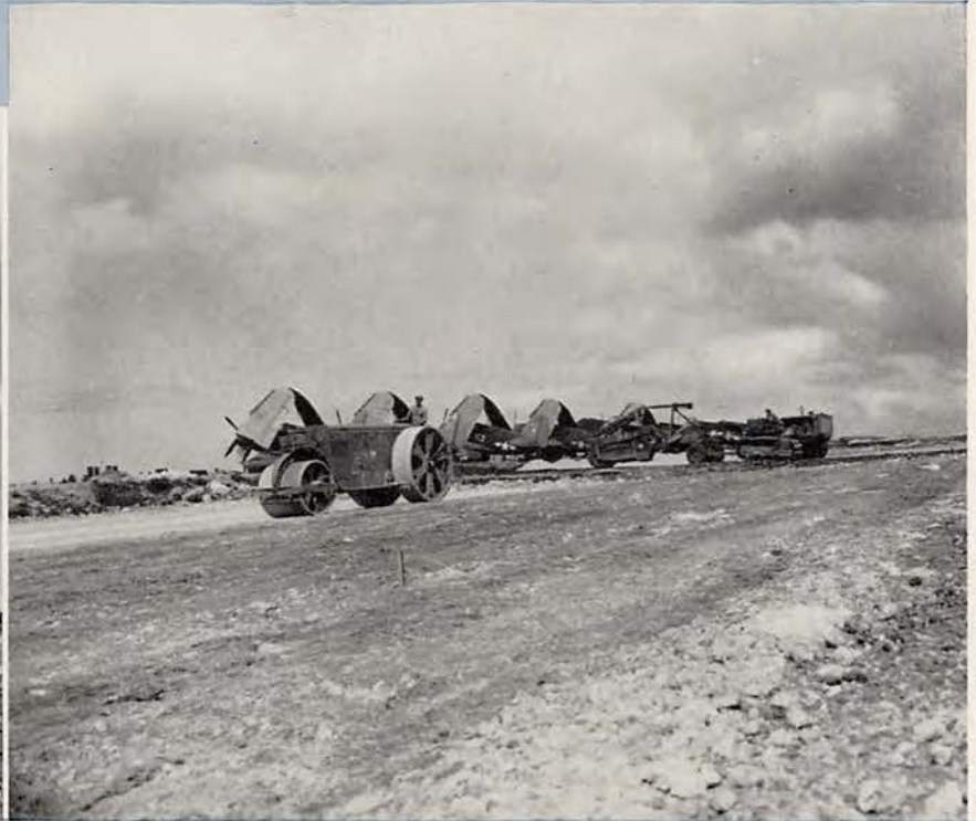
Rolling the hardstands. Bombers will soon be parked here.
