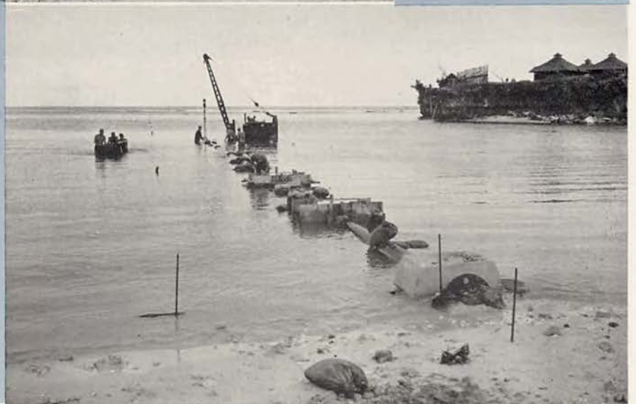
Pouring concrete anchors for sewer outlet.
