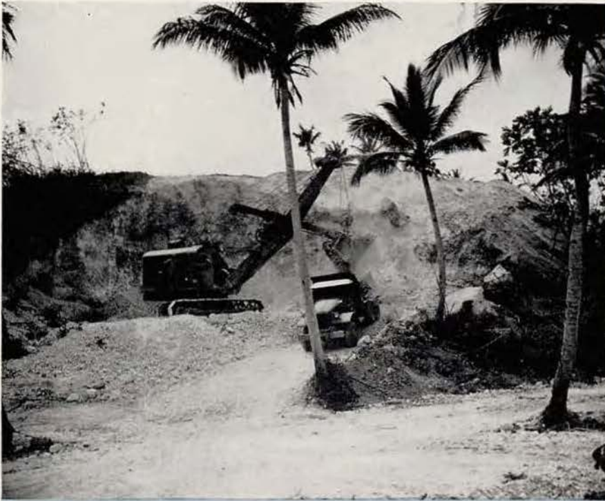
Marianas coral pit. There was no gravel in the Marianas so you substituted coral in the cement mixture.
