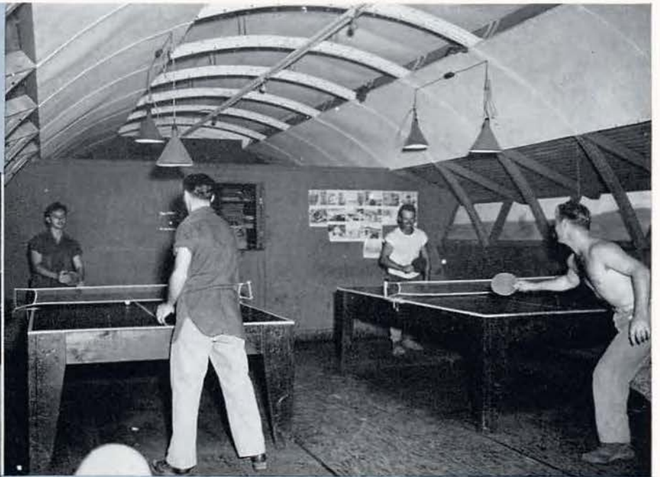
A corner of the Recreation Hut.
