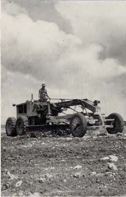
Road scraper leveling earth for airfield hardstands.
