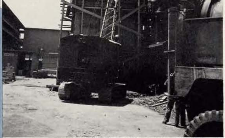
(Below) The exterior completed, crews are cleaning out interior.
