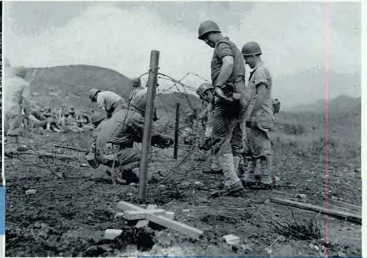
Stringing barb wire.
