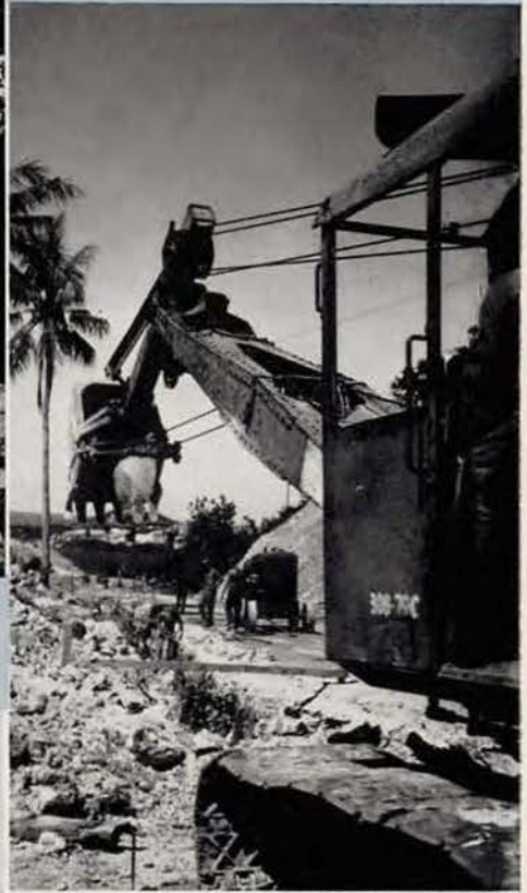
Back hoe, digging a ditch for the sewer line.
