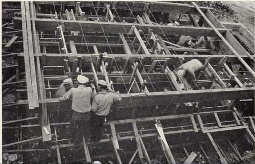
Constructing forms for air compressor foundation.
