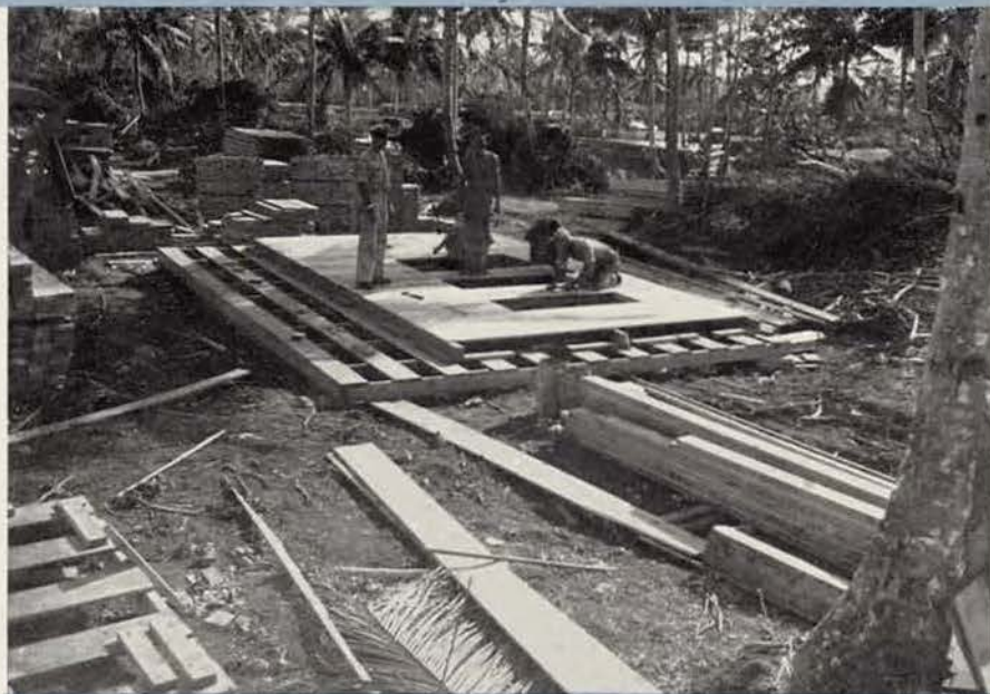
Pre-fabricating warehouses at Marianas airfield.
