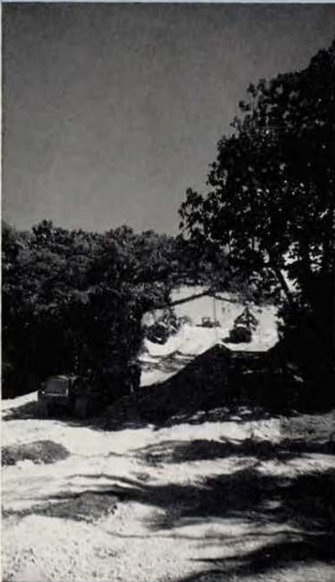
Grading road through coral and jungle.
