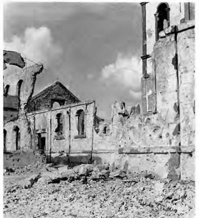
Shells of gutted buildings . .
