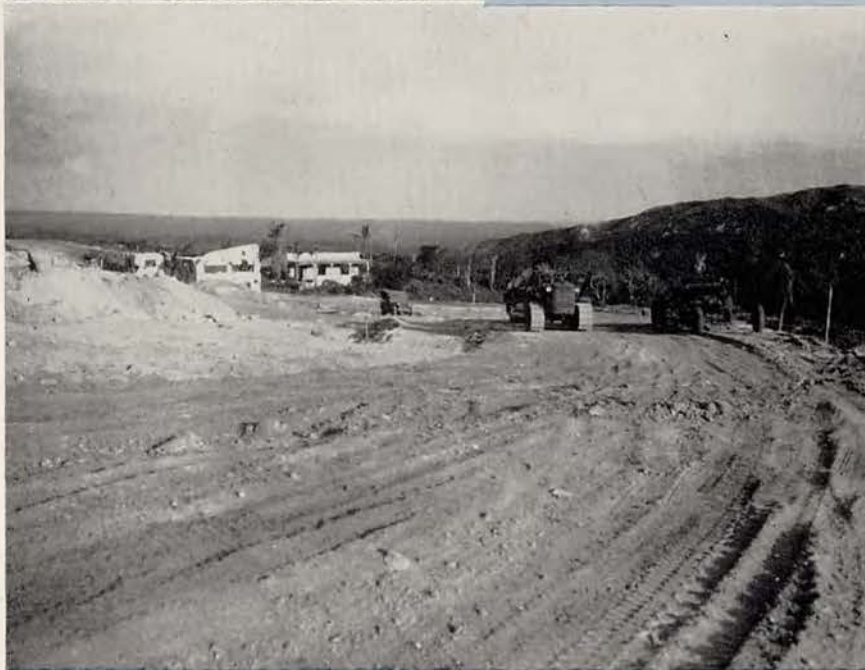
Road grading on Marianas Navy Administration Center job.
