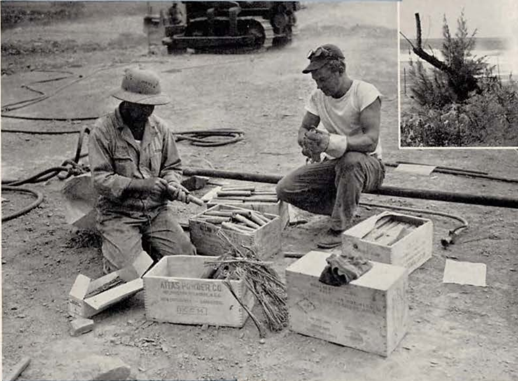
Preparing to set dynamite charge.
