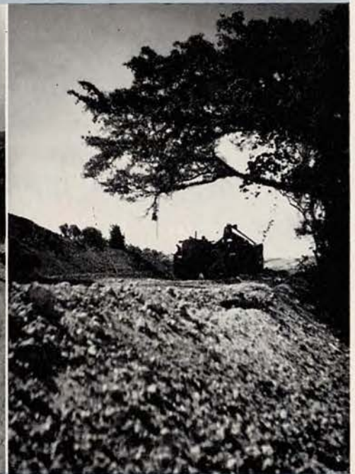
Grading camp road.
