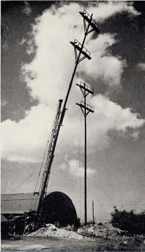
Setting antennae poles for Administration Center radio station.
