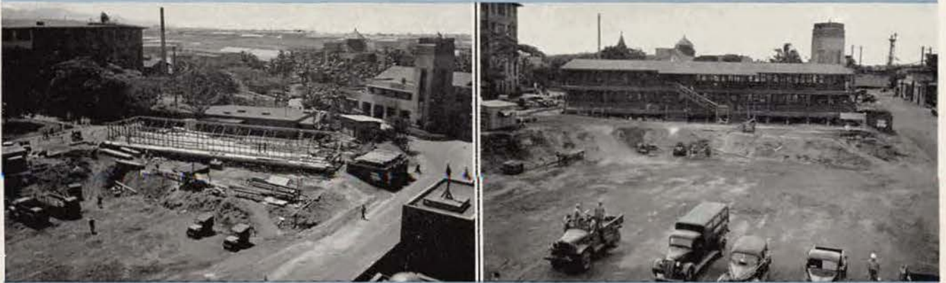
Two construction phases of Sub Base personnel building.
