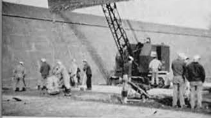
D Co. ON CONCRETE WORK
