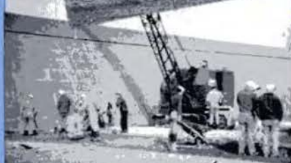
D Co. ON CONCRETE WORK
