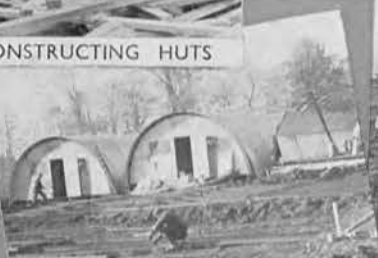
EARLY HUT CONSTRUCTION
