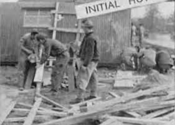
10TH CONSTRUCTING HUTS
