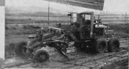
INITIAL WORK ON SIDING
