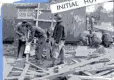
10TH CONSTRUCTING HUTS
