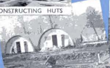
EARLY HUT CONSTRUCTION
