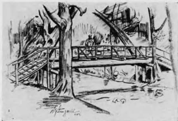
Our first project — a bridge built across a creek in New Caledonia — drawing by H. G. Strugnell, EM2c.
