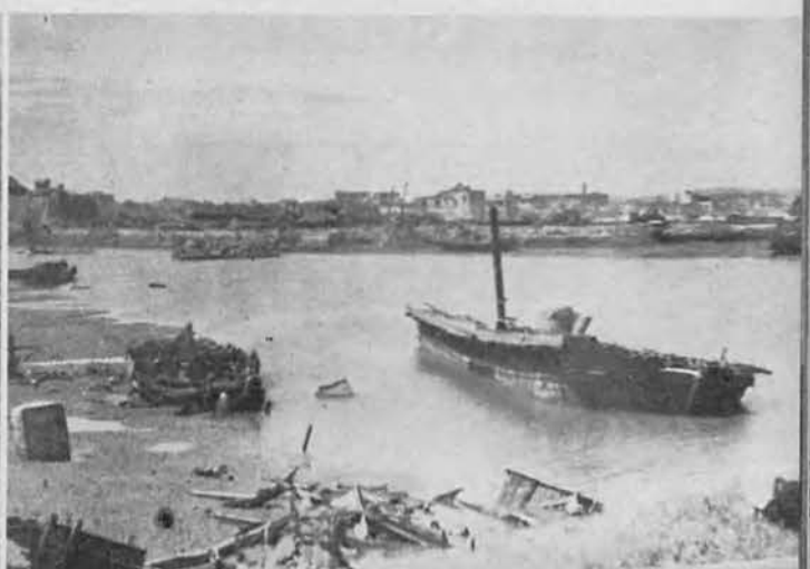
Naba Bay filled with wreckage.
