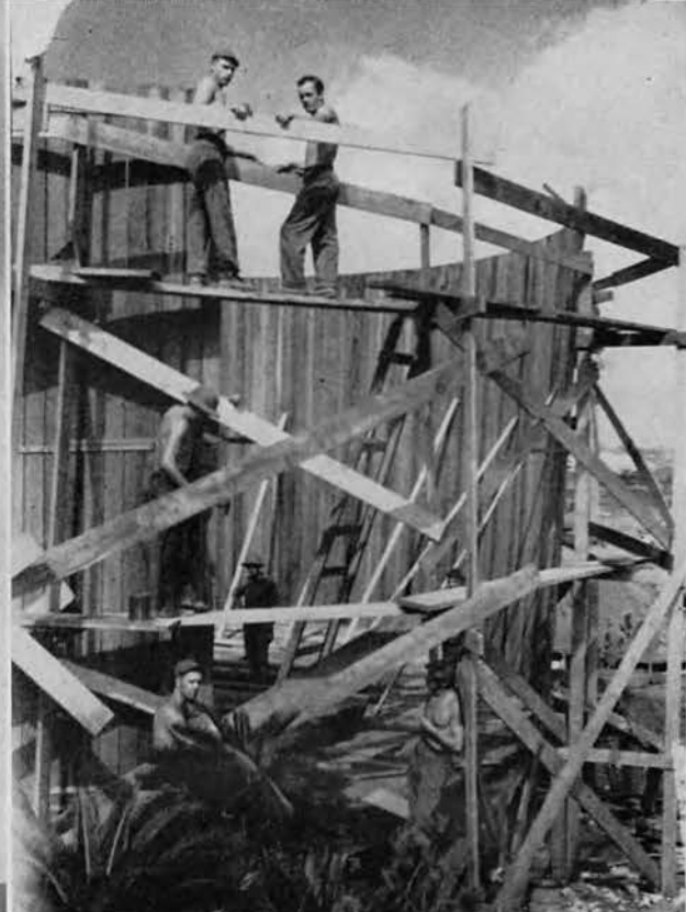
Building a storage tank.
