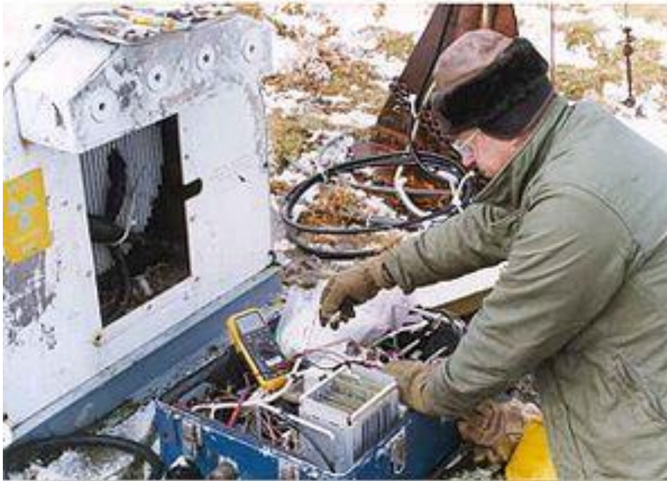
Fairway Rock RTG onsite maintenance.
