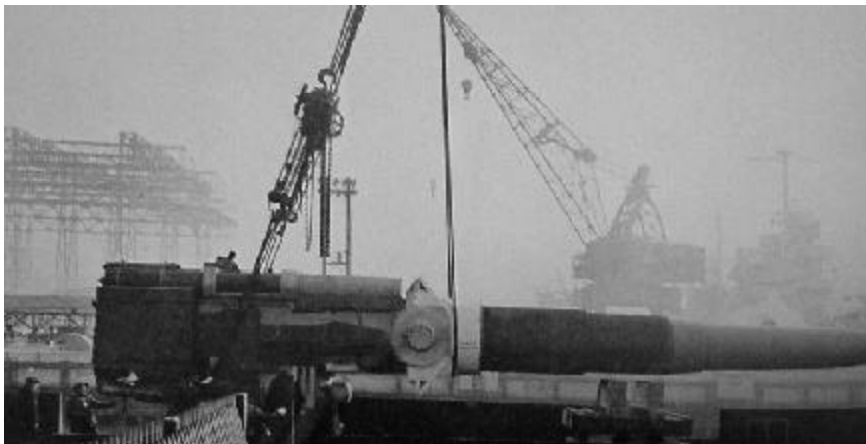
Workers at the Philadelphia Navy Yard prepare to install one of Wisconsin's nine Mk7 16-inch/50-caliber rifles. Manufactured at the Naval Gun Factory at the Washington Navy Yard, the installation of these guns was among the most complicated procedures performed. With the skill of a surgeon, each gun had to be installed within a 1/4-inch of standards. Each gun, not including the gun breech, weighed around 120 tons (considered to be a "lightweight" design) and could fire a one ton shell 24 miles. (U.S. Navy Photo)
