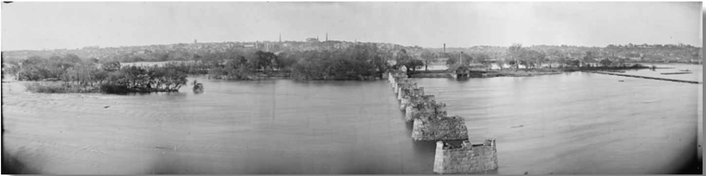
Seen from Manchester, the remains of Mayo's Bridge stretch north to Richmond in this composite of photos made by the Matthew Brady Studio in 1865. (Morgan Riley/National Archives image)
