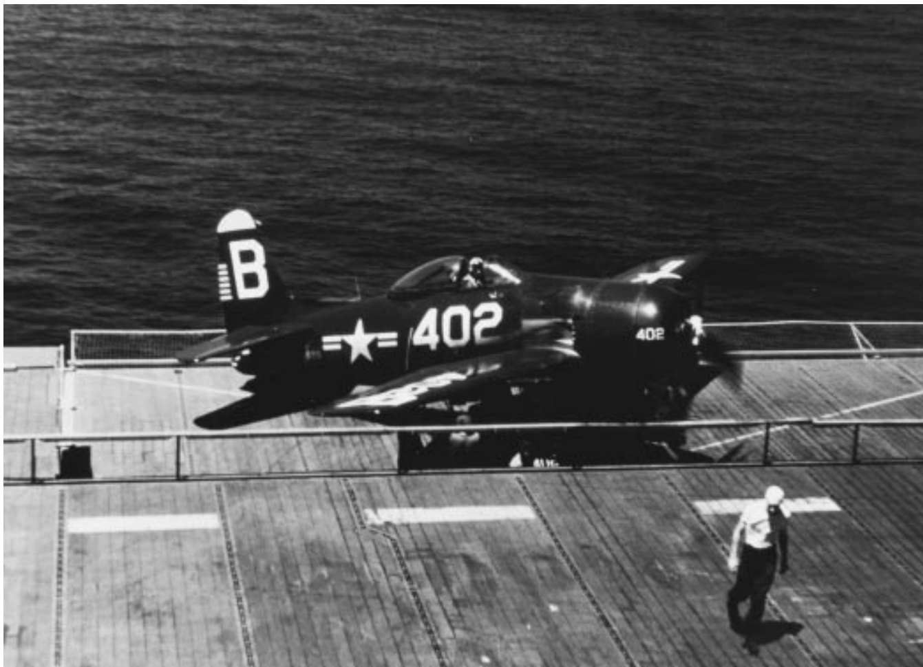
A squadron F8F-2 Bearcat on the elevator being brought up to the flight deck, 1950 (Courtesy Robert Lawson Collection).
