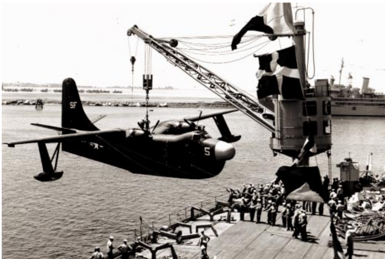
A squadron P5M being hoisted aboard a seaplane tender.
