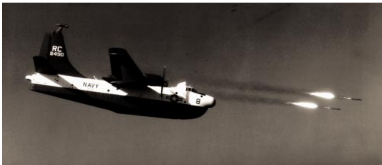
A squadron P5M launching missiles (HVAR, 5 inch High Velocity Aircraft Rockets).
