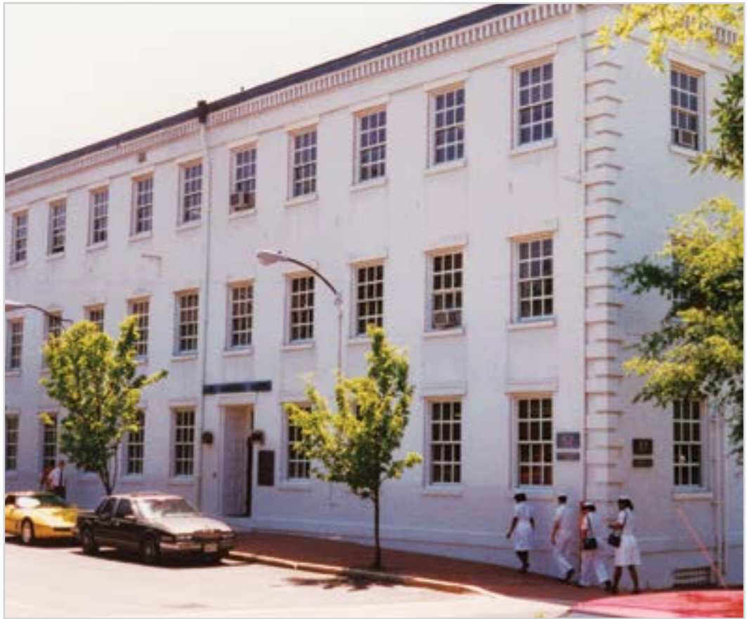
The Dudley Knox Center for Naval History (Building 57).
