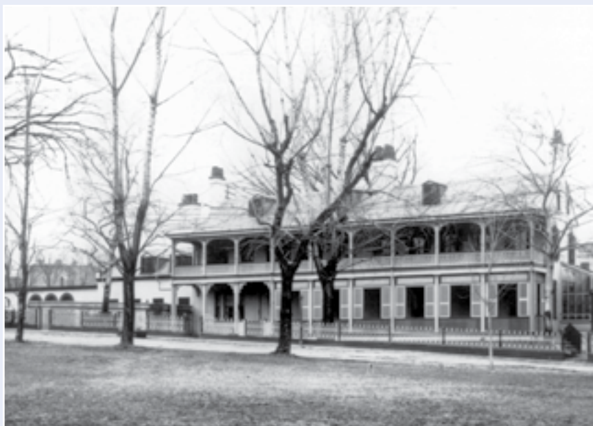
Quarters B or Second Officer's Quarters, the oldest structure at the Washington Navy Yard. Early in the 19th century, local builders Lovering and Dyer created this residence for officers who served as second in command at the naval facility. The building later served as a barrack for the U.S. Marine guard force and then the residence of the Commandant, Naval District Washington.
