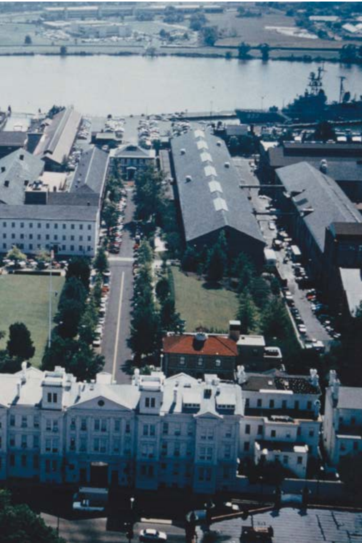
An aerial view of the navy yard in 1998. Visible in the foreground are Latrobe Gate, the rear of Tingey House, and Leutze Park. Decommissioned destroyer Barry (DD 933) is moored on the Anacostia River waterfront.
